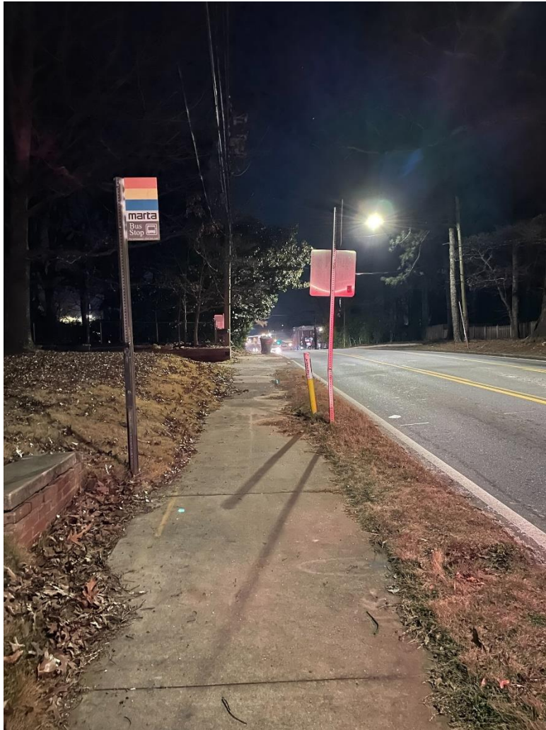
Figure 9 - Example of Adequate Intersection Lighting along SR 154 / Memorial Dr
