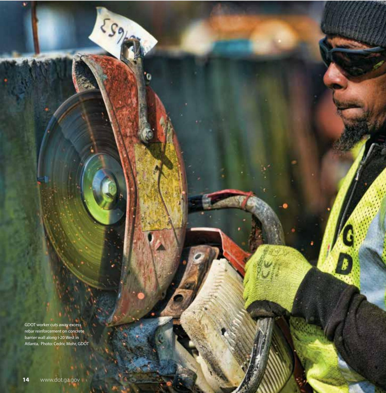
GDOT worker cuts away excess rebar reinforcement on concrete barrier wall along I-20 West in Atlanta. Photo: Cedric Mohr, GDOT
