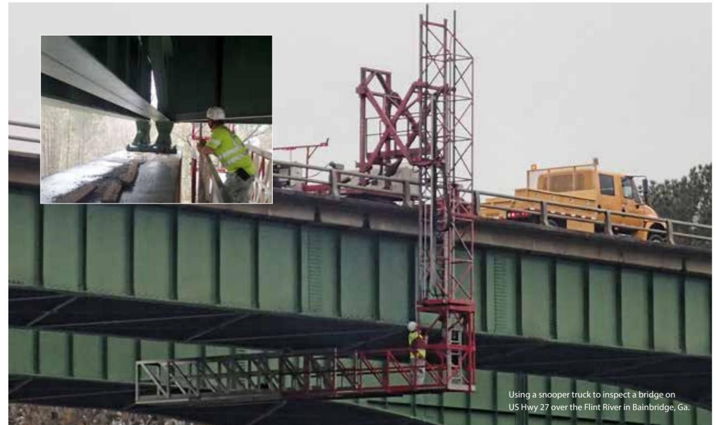
Using a snoopercrane to inspect a bridge on US Hwy 27 over the Flint River in Bainbridge, Ga.
