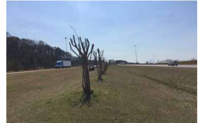
**Bioswales.** The Ray and the Georgia Department of Transportation installed five acres of native grasses and pollinator plant seeds in the median and northbound lane gore area of Exit 6 on I-85 near LaGrange. These areas, known as bioswales, are shallow drainage ditches filled with vegetation to slow water movements and capture particulate pollutants, heavy metals, rubber and oil during rainstorms. Photo: The Ray
