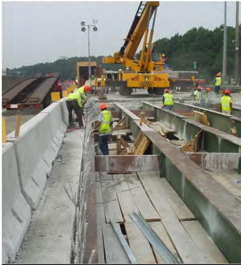
Construction crews working on bridge deck reconstruction
