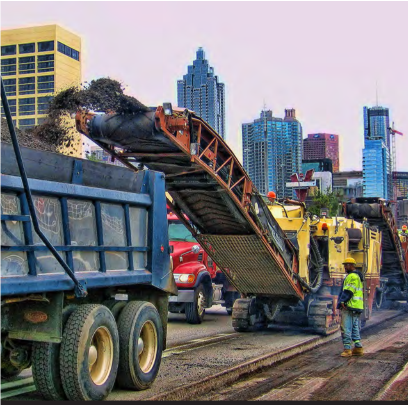
Crews perform milling and inlay work
