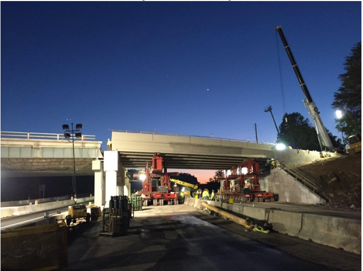
I-24 at SR 299 Bridge under construction during 56 hour move
