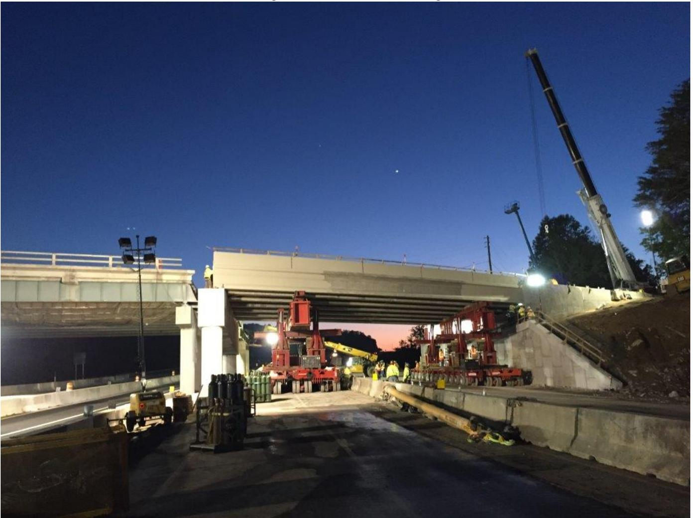
1. **Project Description:** The proposed project [P.I. No. 0011682] replaced the existing, structurally deficient State Route (SR) 299 bridge over Interstate 24 (I-24) in Dade County, Georgia. This overpass is approximately 0.6 miles south of the Georgia/Tennessee state line at the I-24 Exit 169 interchange. The bridge was replaced on the existing alignment using Accelerated Bridge Construction (ABC) techniques.
