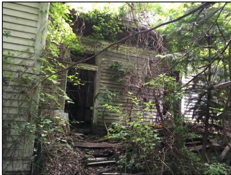
Image 10. Abandoned house with potential to serve as a summer roost site
