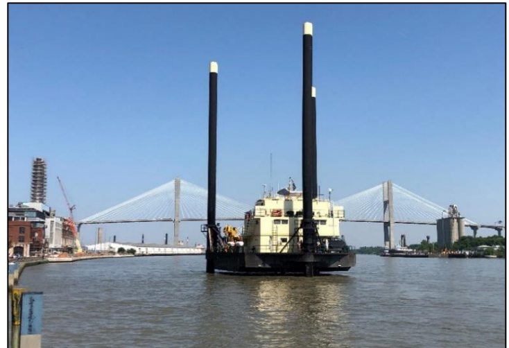
Photo 3. Barge setup in an open water during a GDOT project drilling event. Source: Terracon
