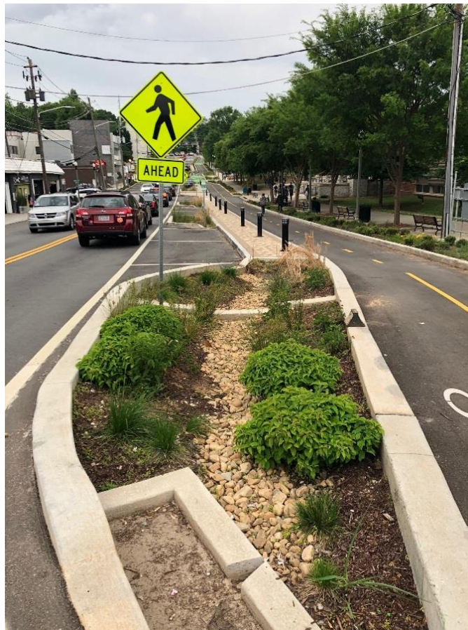
Figure 6.28. Example of Green Infrastructure, Decatur, Georgia
