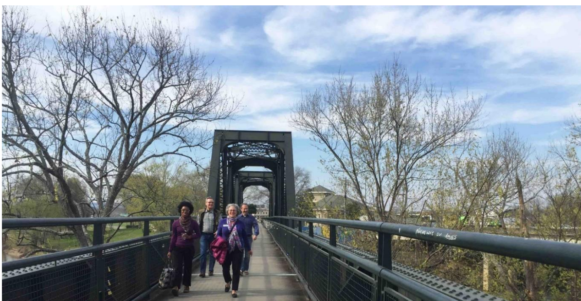
Figure 4.411. Retrofitted Train Trestle Pedestrian Bridge, Rome, Georgia
