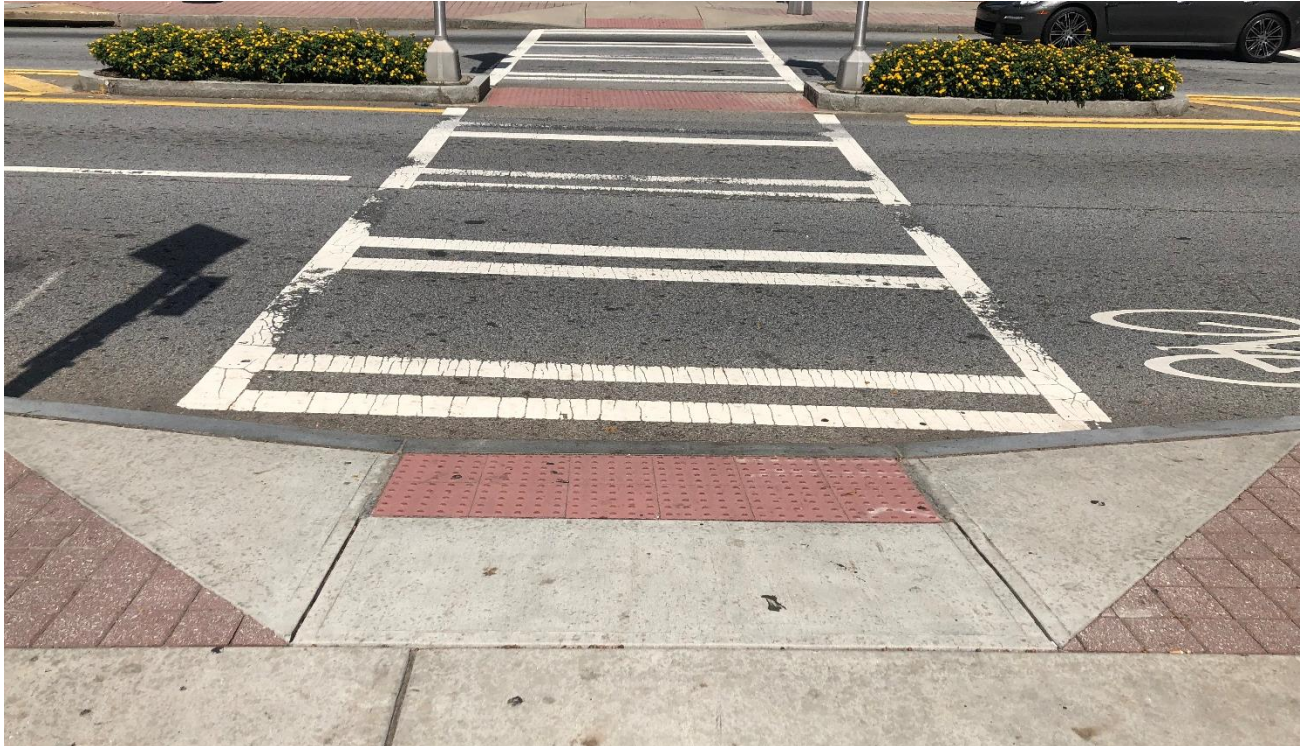
Figure 4.35. Example of Curb Ramp
