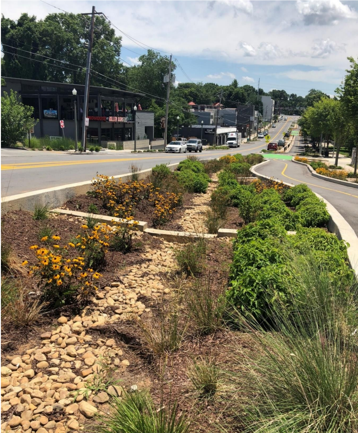
Figure 6.29. Example of Green Stormwater Infrastructure, Decatur, Georgia
