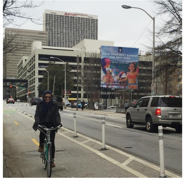
Figure 6.16. Example of Flexible Bollards
