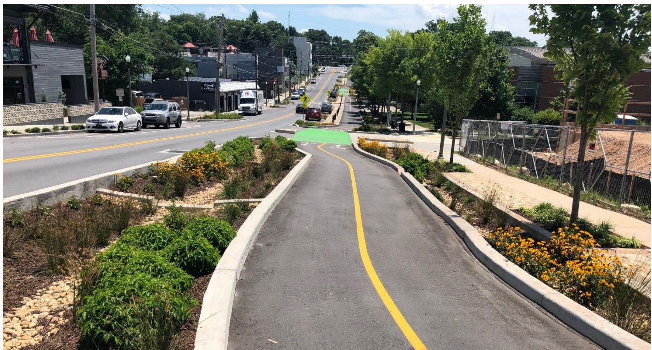
Figure 4.12. Two-Way Buffered Cycle Track with Green Infrastructure, Decatur, Georgia
