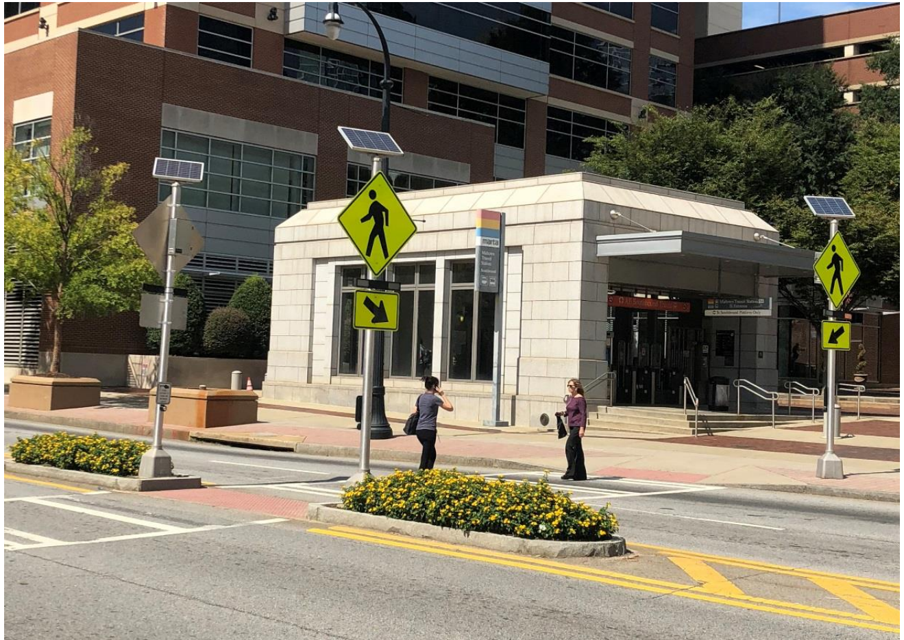
Figure 4.17. Mid-Block Crossing with Pedestrian Refuge Area, Atlanta, Georgia
