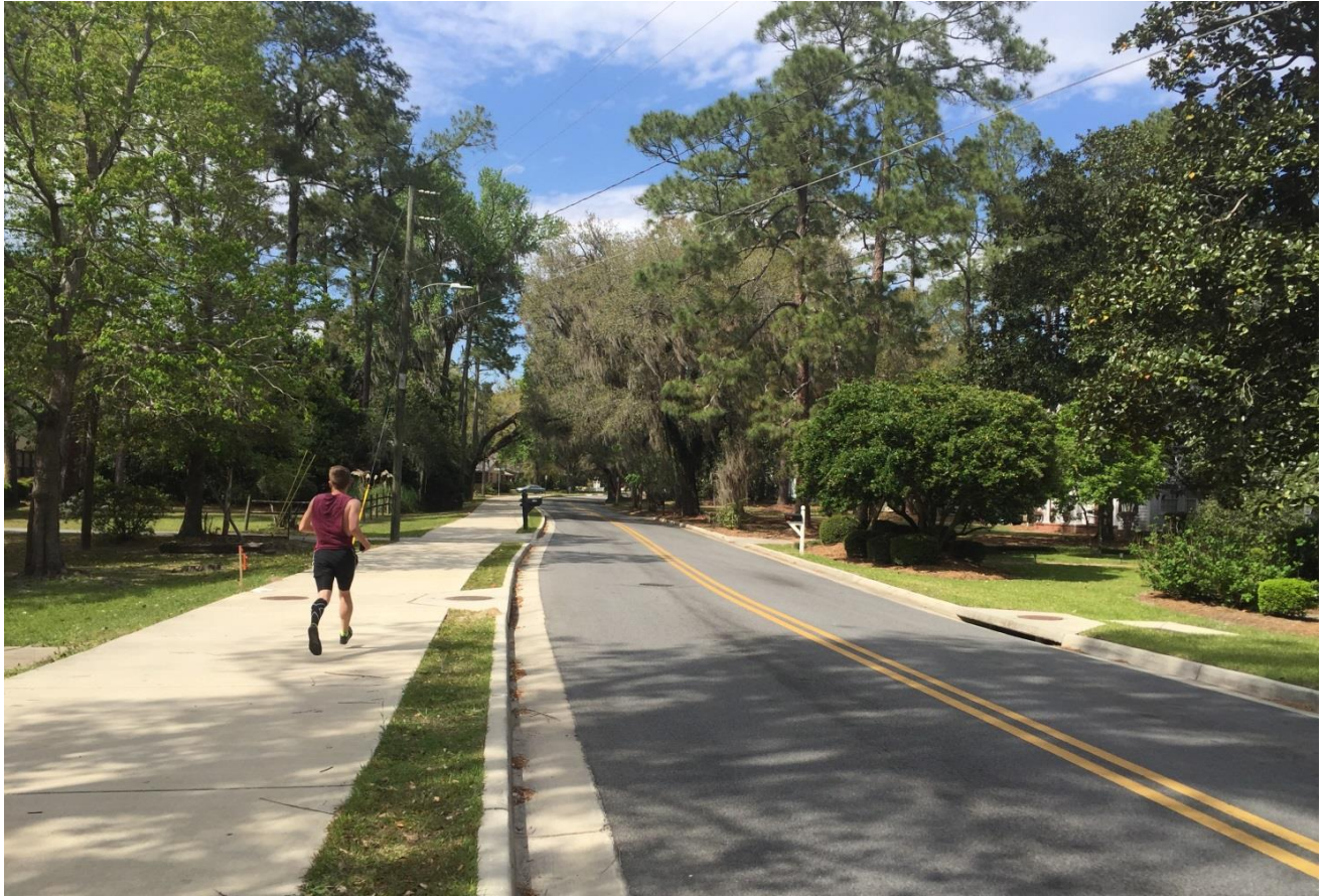
Figure 4.22. Azalea Trail Shared Use Path on Street with speeds less than 35 mph, Valdosta, Georgia
