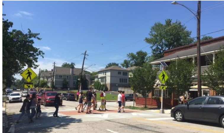
Figure 3.1. Raised Crosswalk with RRFBs, Atlanta, Georgia
