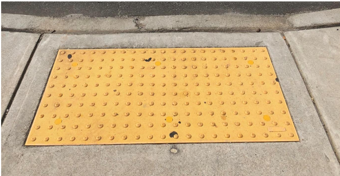
Figure 4.10. Detectable Pavers – “Safety Yellow”
