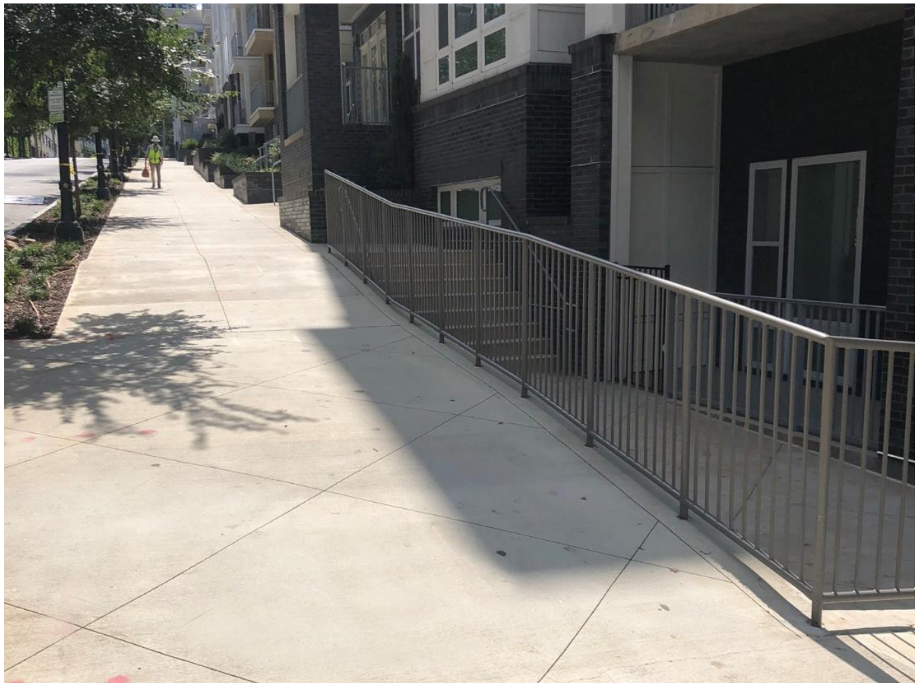
Figure 4.13. Pedestrian Safety Railing, Midtown, Atlanta, Georgia
