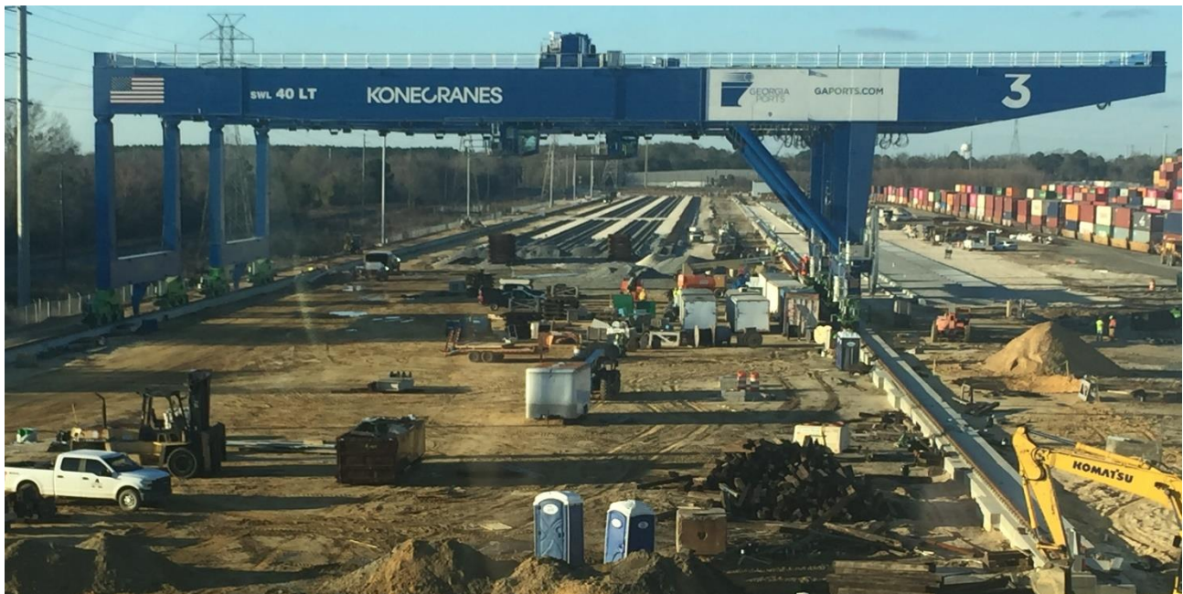
Figure 4-7: Mason Mega Rail Yard under Construction January 2020
