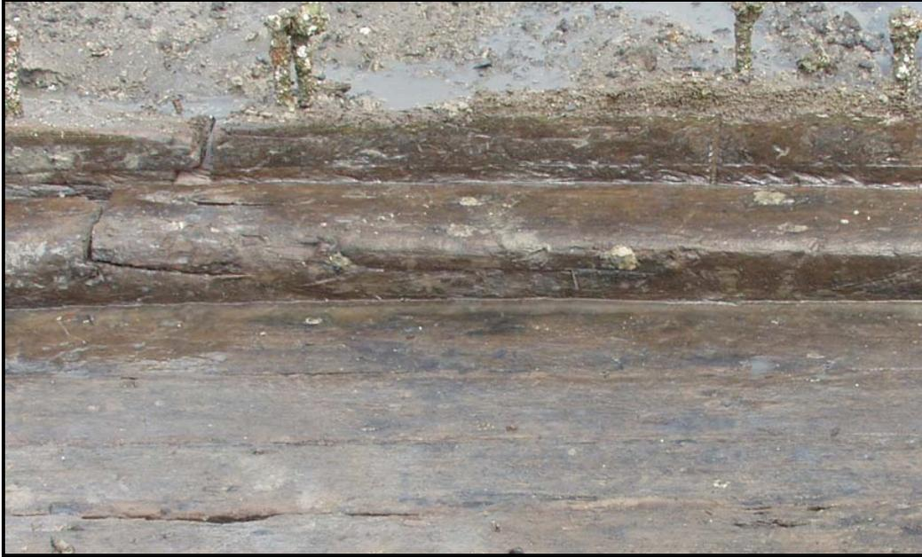
**Figure 53. Bilge ceiling, keelson, rider keelson and starboard sister keelson showing scarfs and fastening pattern.**
