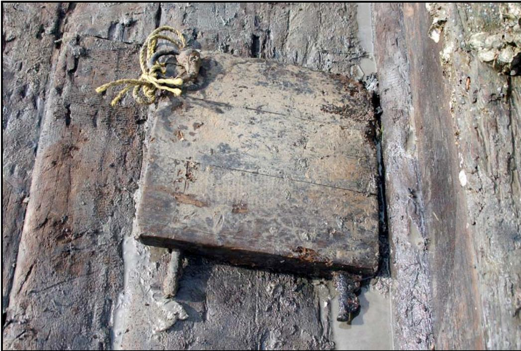
**Figure 66. Hatch for lumber port.**
