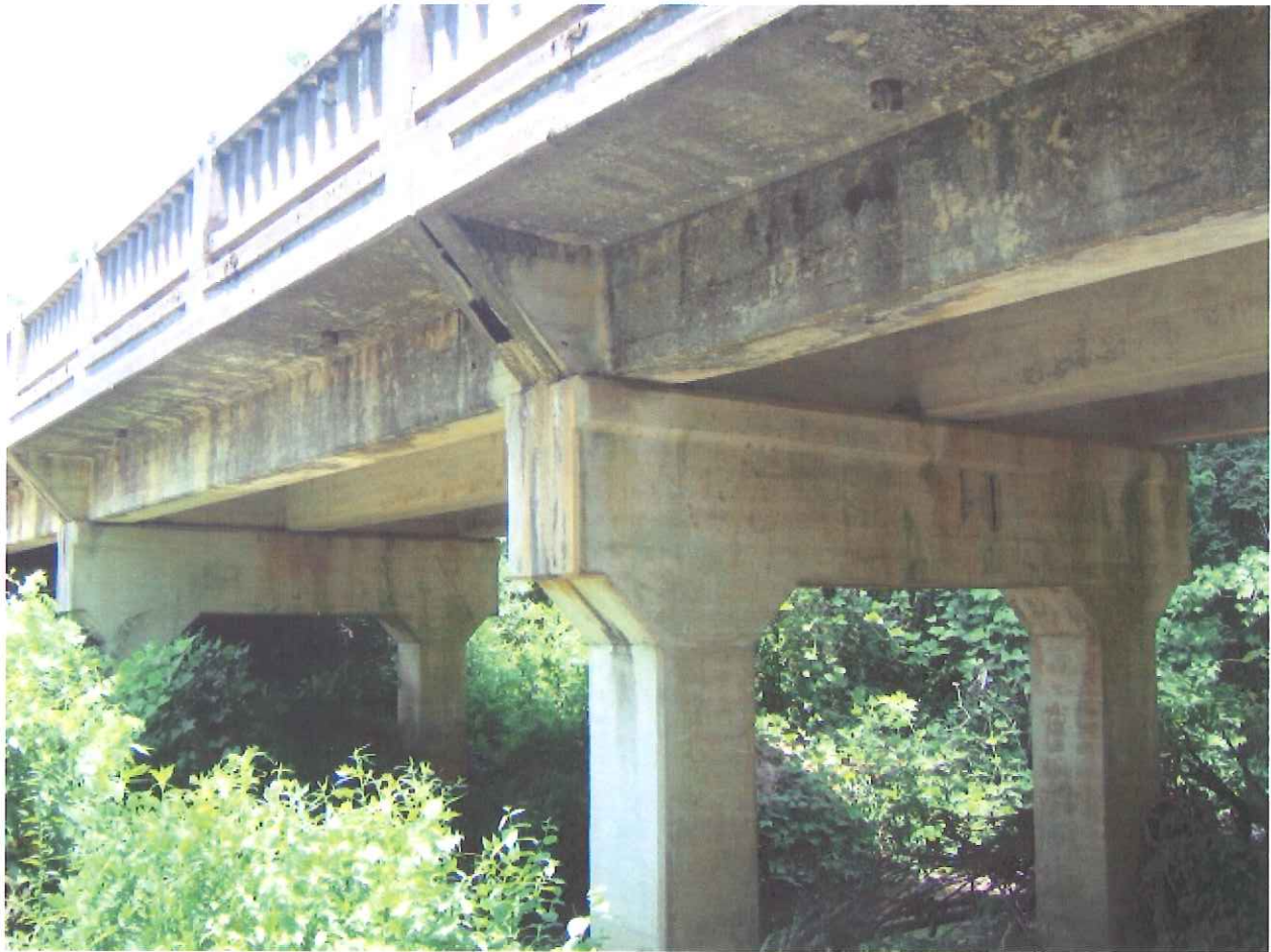
Rabun County, GDOT Bridge #241-5027-0, CR 153 at Tiger Creek, 1926
