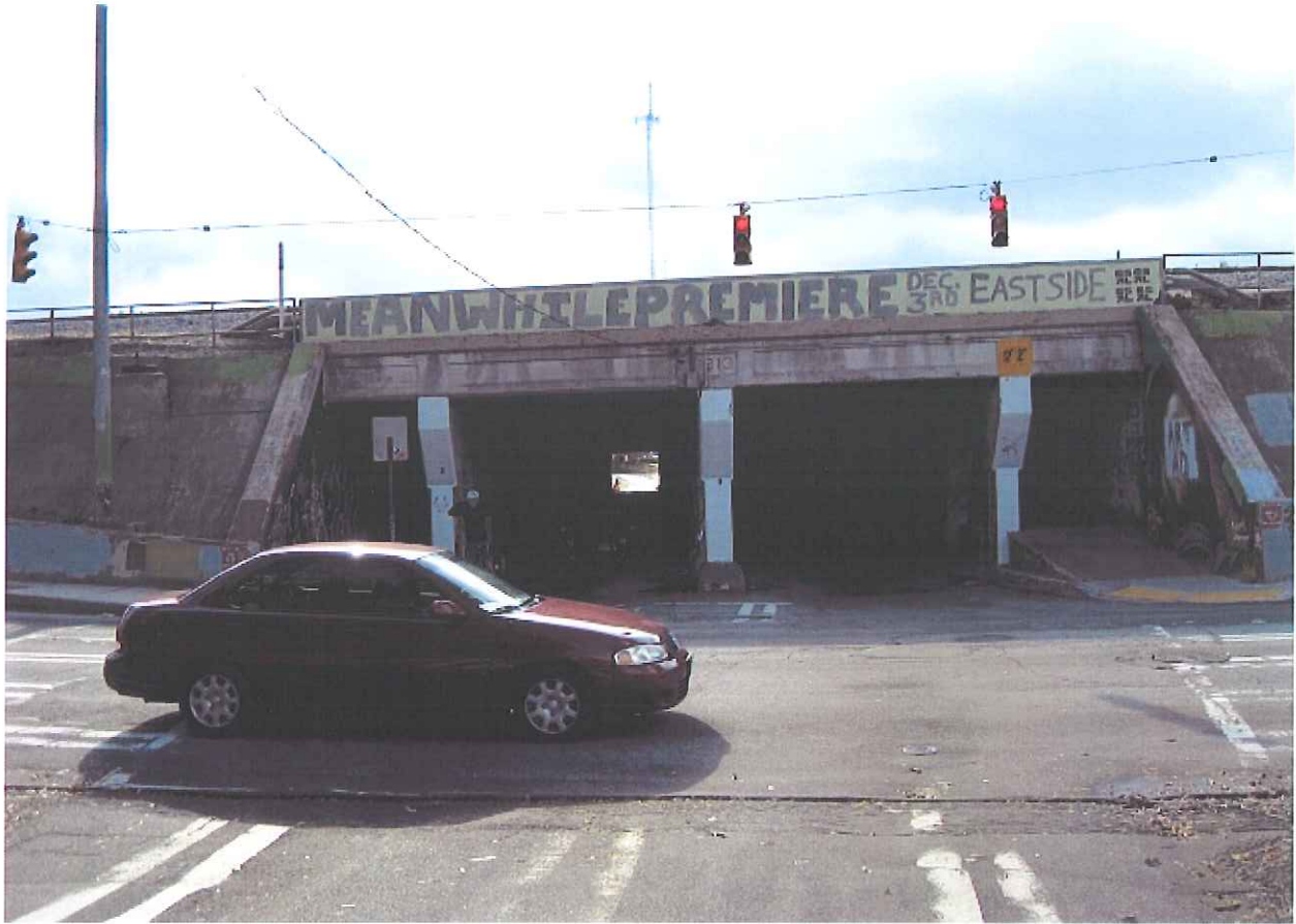
Fulton County, GDOT Bridge #121-5148-0, CSX RR over Estonia Drive, 1913
