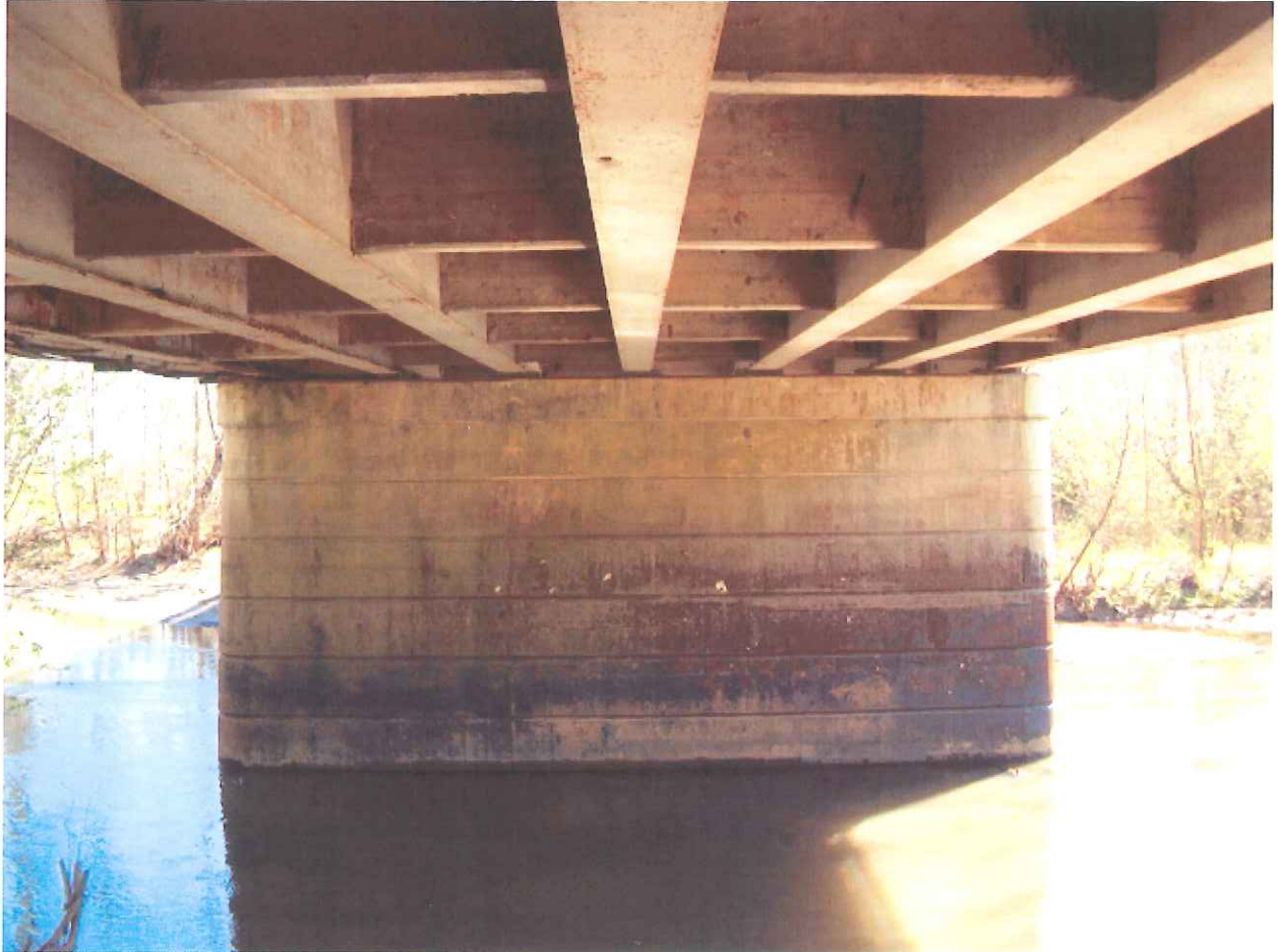
Bibb County, GDOT 021-0182-0, Jeffersonville Road at Walnut Creek, 1929
