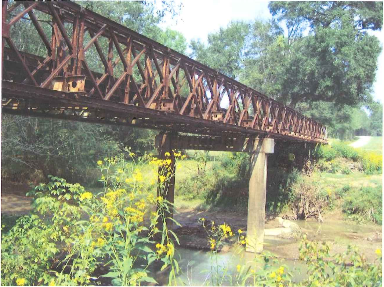
Murray County, GDOT Bridge #213-5007-0, Old Federal Road at Mill Creek, 1918
