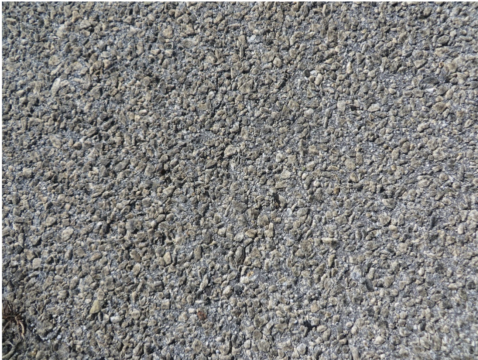
TAWI-10. Weathering (Sample Unit No. 45).
