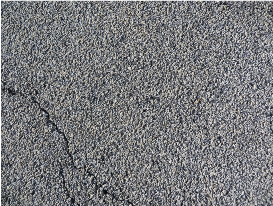
R523WI-20. Weathering (Sample Unit No. 02).
