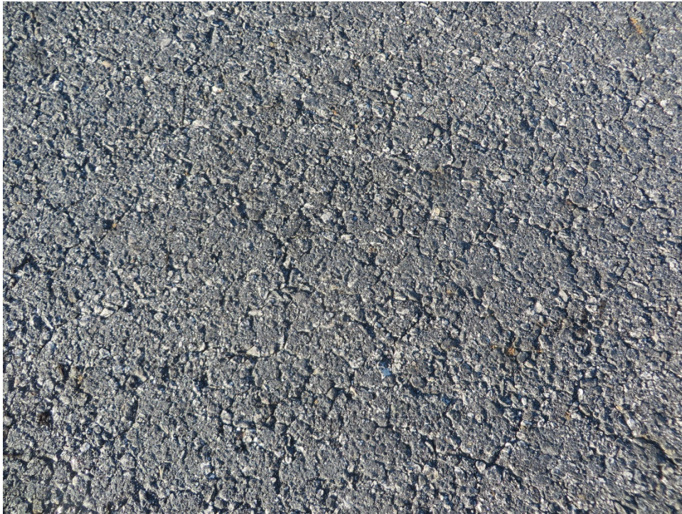
A01WI-20. Weathering (Sample Unit No. 02).
