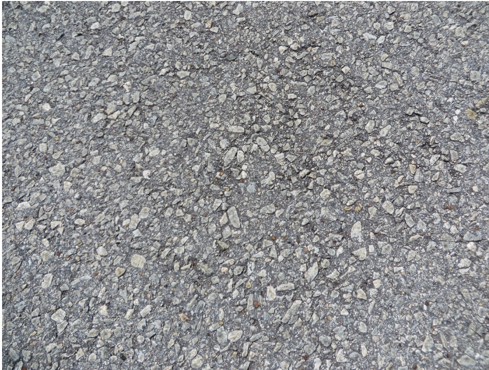
THANGWI-20. Weathering (Sample Unit No. 17).
