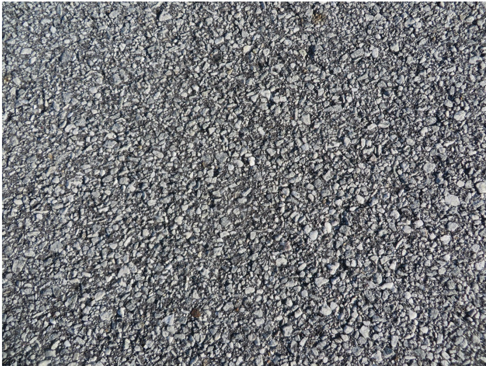
R523WI-10. Weathering (Sample Unit No. 04).
