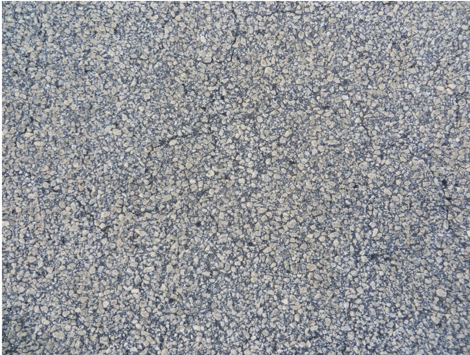
TDWI-30. Weathering (Sample Unit No. 01).
