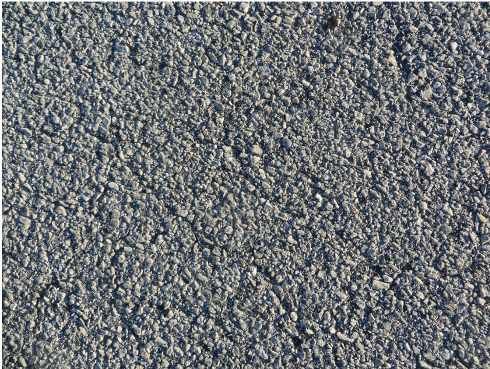
A01WI-10. Weathering (Sample Unit No. 30).
