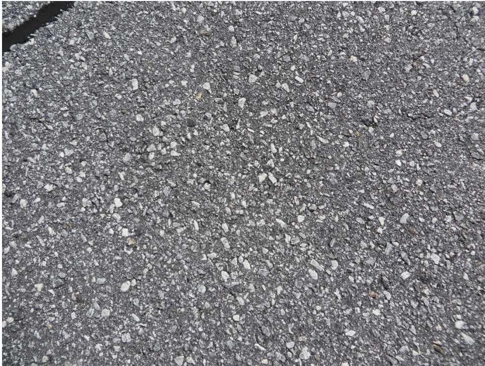
TDWI-10. Weathering (Sample Unit No. 22).
