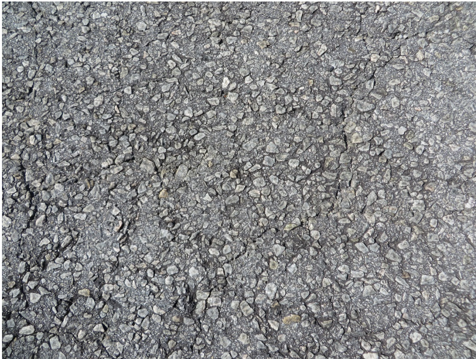
THANGWI-10. Weathering (Sample Unit No. 02).
