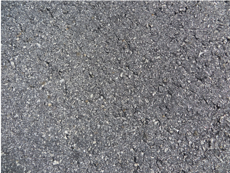
A02WI-20. Weathering (Sample Unit No. 01).
