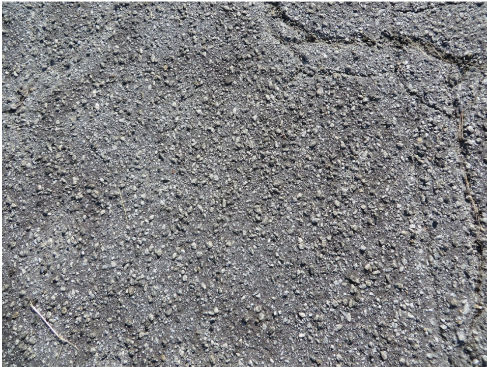
A02WI-10. Weathering (Sample Unit No. 03).
