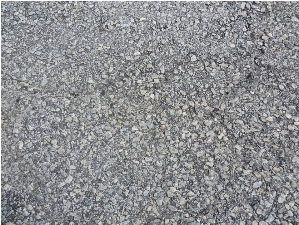
TDWI-20. Weathering (Sample Unit No. 01).
