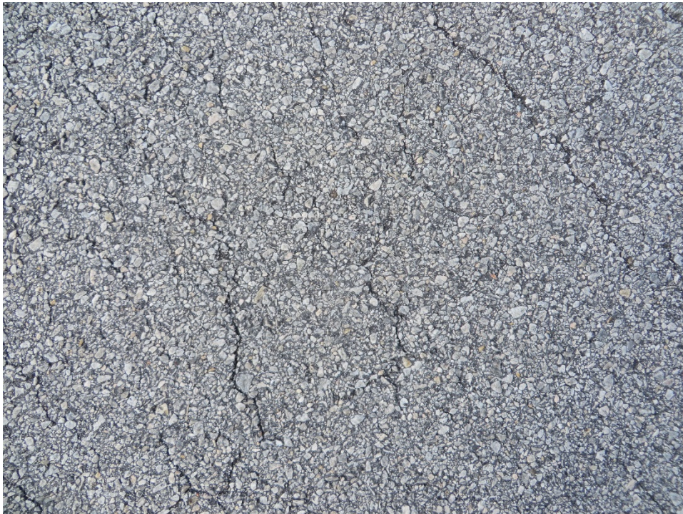
THANGWI-30. Weathering (Sample Unit No. 02).
