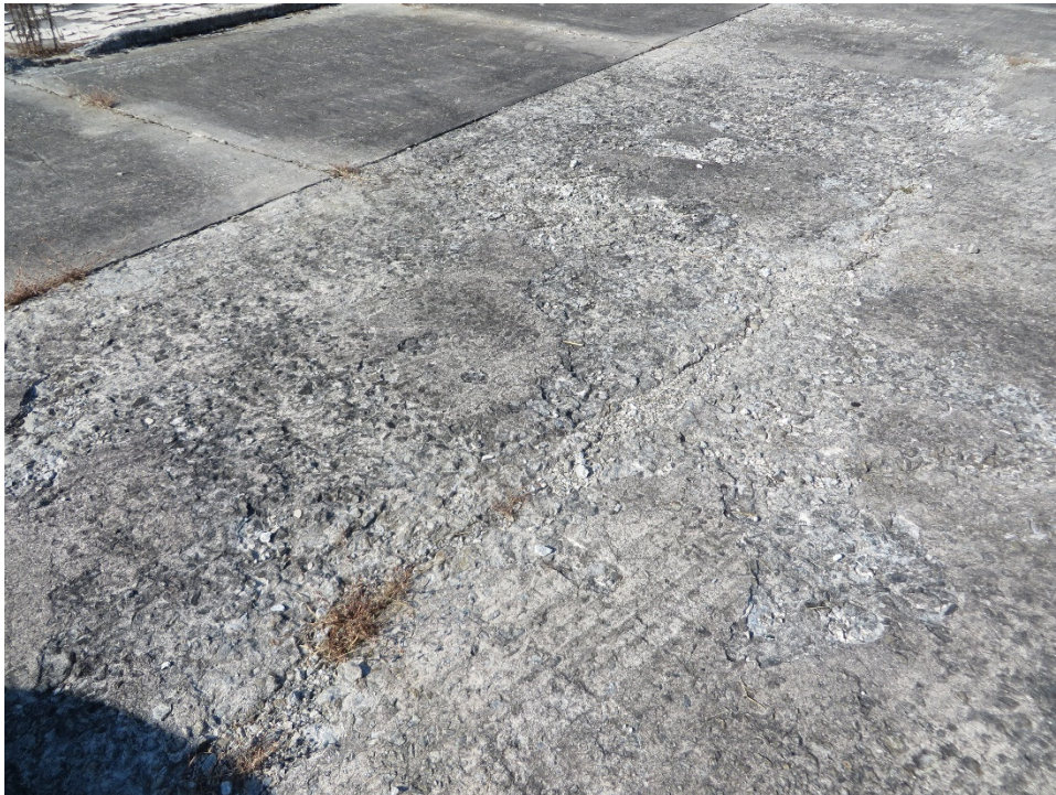
A02WI-30. Scaling (Sample Unit No. 02).
