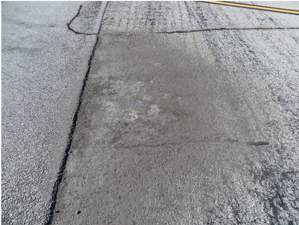
THANGML-10. Depression (Sample Unit No. 01).
