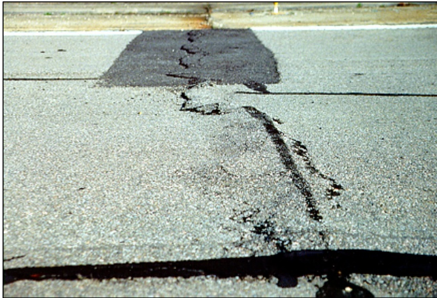
FIGURE H-9 HIGH-SEVERITY SWELLING
