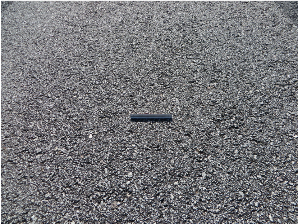
R1735ML-10. Weathering (Sample Unit No. 02).
