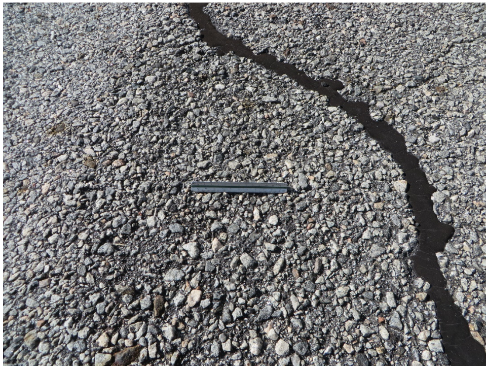
THANGML-10. Raveling (Sample Unit No. 05).
