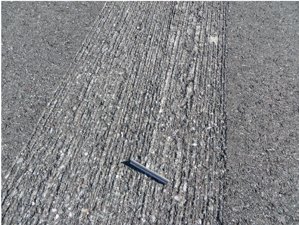
R1432HO-20. Weathering (Sample Unit No. 12).
