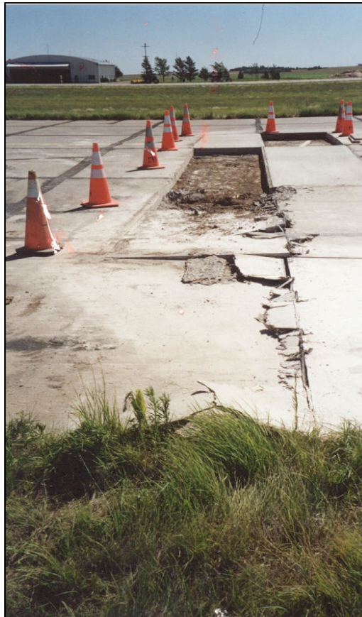
FIGURE H-10 HIGH-SEVERITY BLOWUP IN THE PROCESS OF BEING REPAIRED
