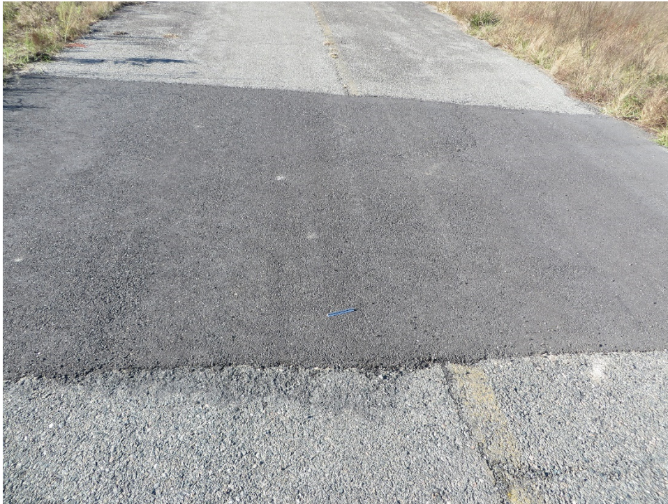
TAHO-10. Patching (Additional Sample Unit No. 02).
