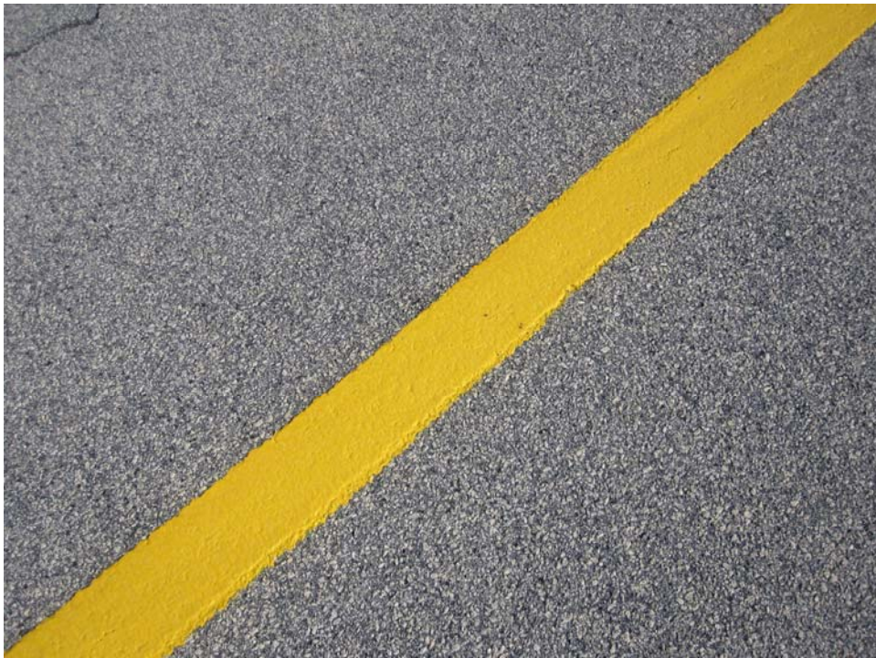
TAWB-10. Satisfactory Paint.
