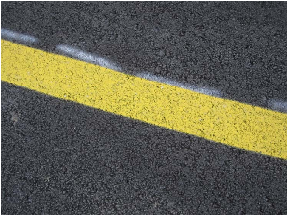
TAML-10. Satisfactory Paint.
