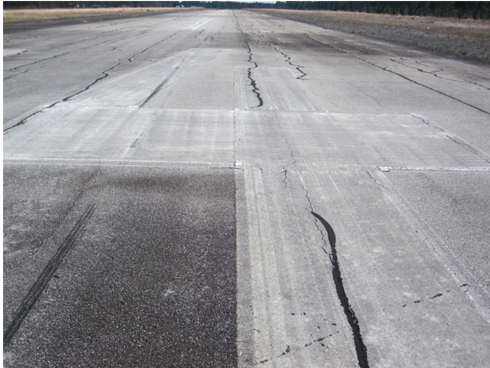
R1432HO-10. Unsatisfactory Paint.
