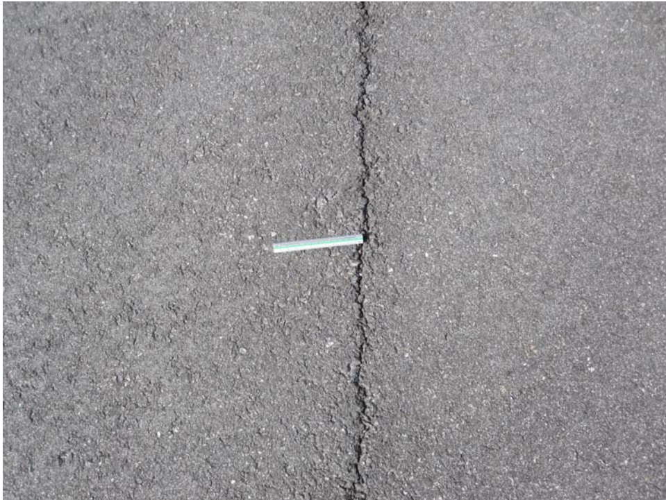
TBAL-30. Longitudinal and Transverse Cracking (Sample Unit #03).
