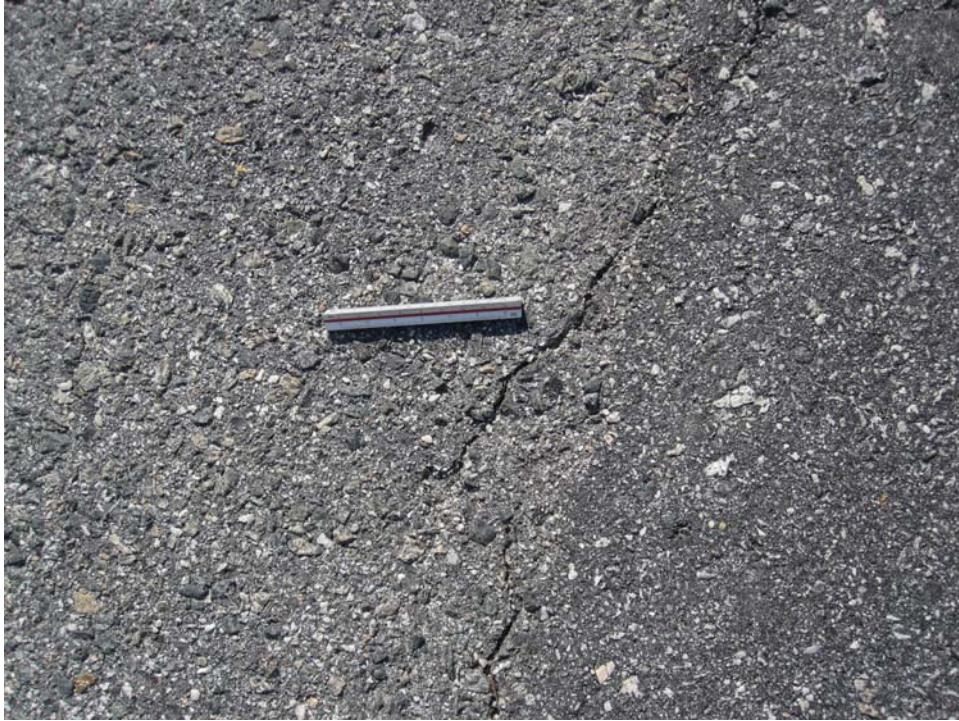
THANGAL-10. Longitudinal and Transverse Cracking (Sample Unit #03).
