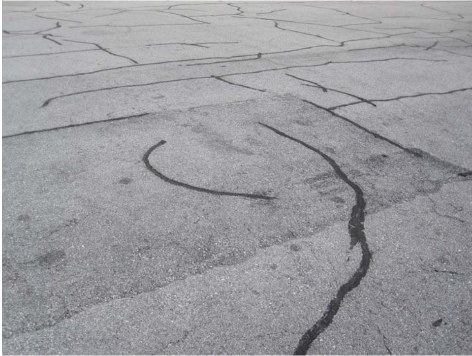
A01AL-10. Patching (Sample Unit #09).
