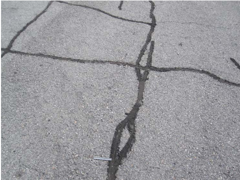
A01AL-10. Block Cracking (Sample Unit #01).
