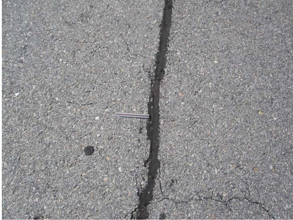
TAAL-10. Longitudinal and Transverse Cracking (Sample Unit #01).
