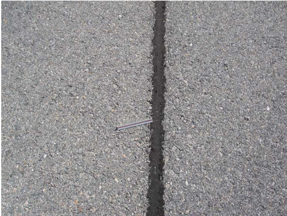
R1533AL-10. Longitudinal and Transverse Cracking (Sample Unit #95).
