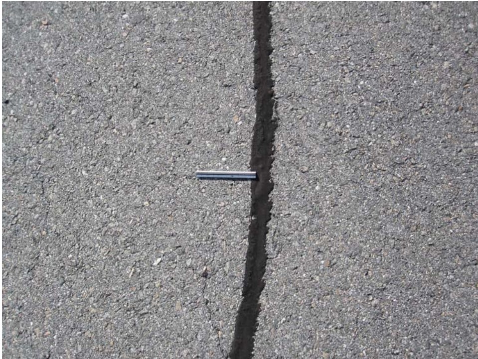
TBAL-10. Longitudinal and Transverse Cracking (Sample Unit #01).
