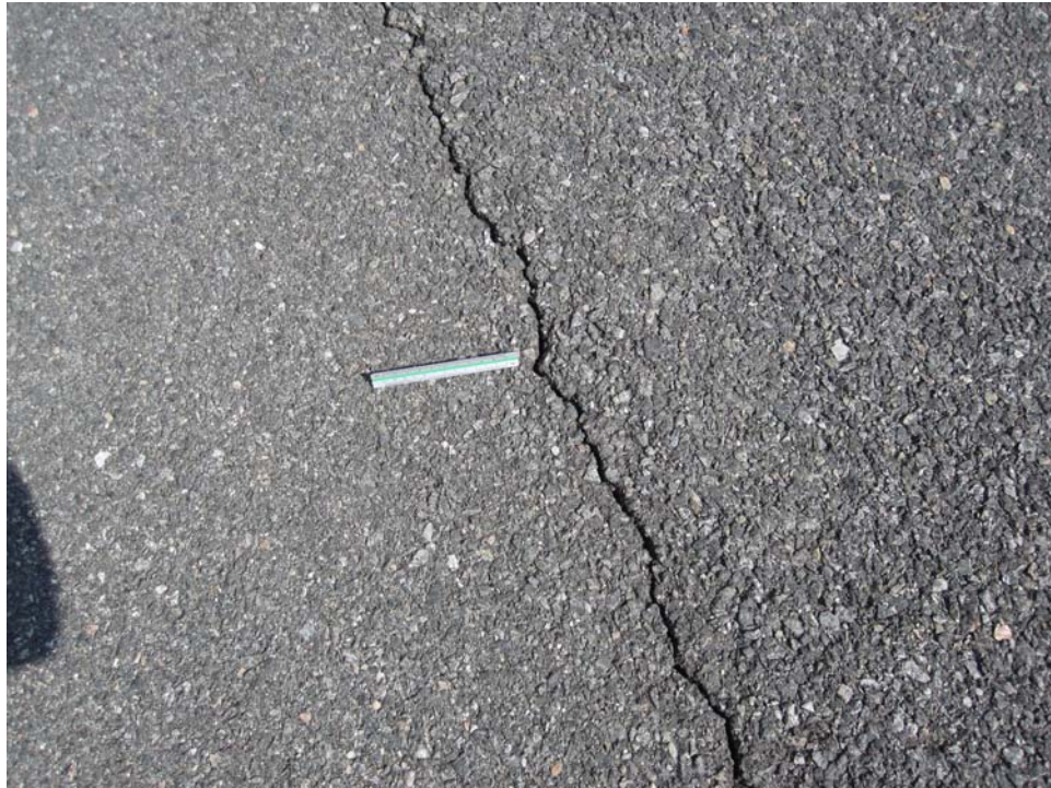
TBAL-20. Longitudinal and Transverse Cracking (Sample Unit #01).
