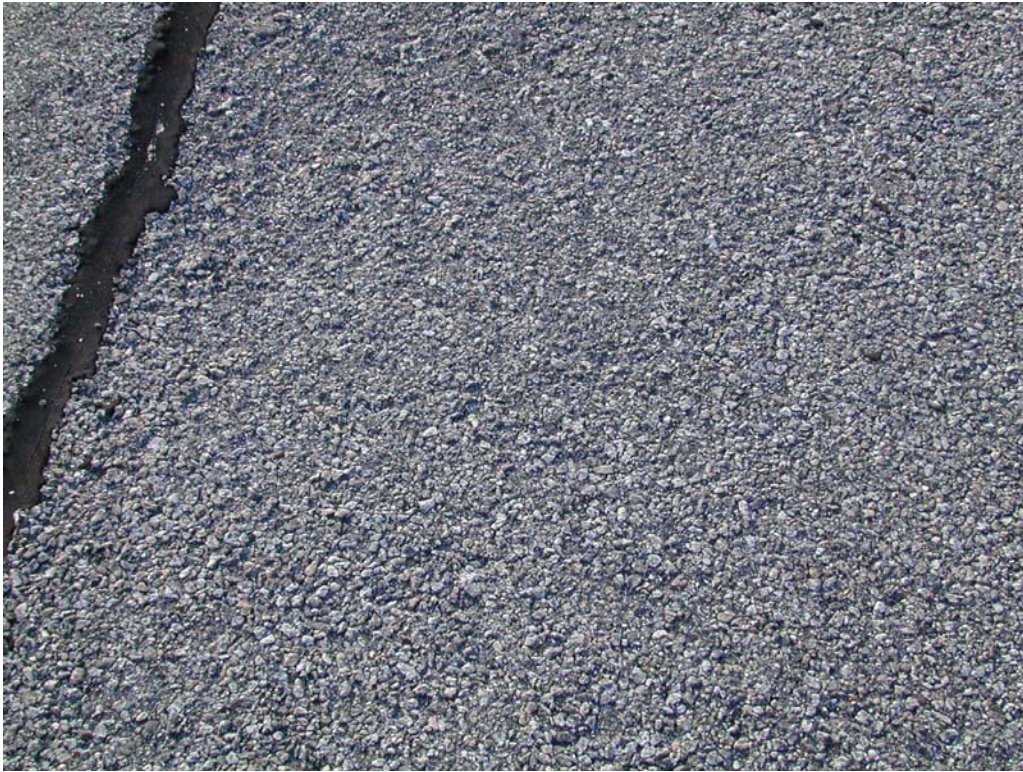
Raveling and weathering in section TAML-10.
