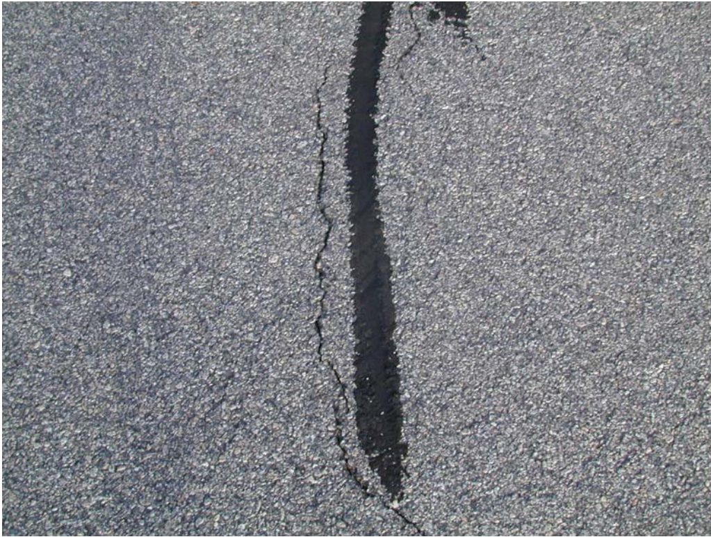
L&T cracking in section A01ML-10.
