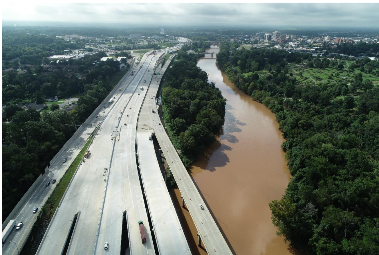
Photo: Northbound Interstate-75 at Interstate-16, Macon Cover Photo: Interstate-75 South of Macon to Interstate-75 West of Bolingbroke Boling
