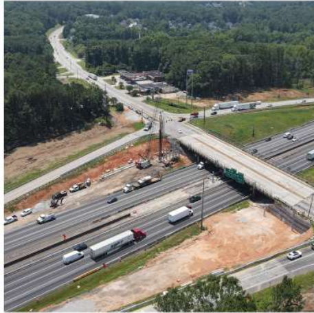
Currently under construction, the project will consist of the reconstruction of the I-285/Bouldercrest Rd interchange including the replacement of the Bouldercrest Rd bridge. The new bridge will consist of six 12-foot travel lanes and six-foot sidewalks with four-foot bike lines for both directions of travel along Bouldercrest Rd. Image taken by District 7 UAS Pilot Jakari Dean.
