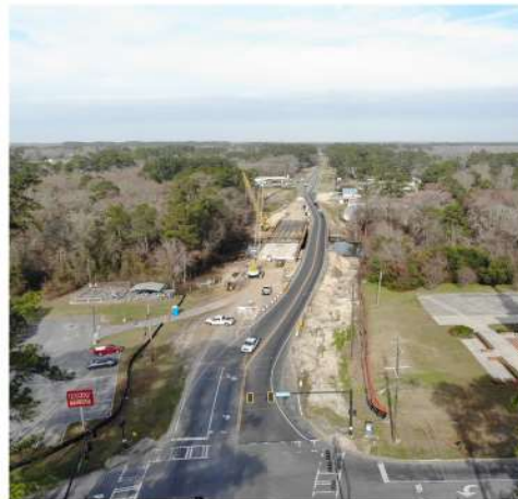
The project consists of 8.5 miles of road widening and relocation on SR 133 in Colquitt County. This Bridge is 450 feet long with 30-foot approach slabs on both sides over the Okapilco Creek North of Moultrie. Images taken by District 4 UAS Pilot Courtney Joseph Peugh.
