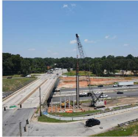
Currently under construction, the project will consist of the reconstruction of the I-285/Bouldercrest Rd interchange including the replacement of the Bouldercrest Rd bridge. The new bridge will consist of six 12-foot travel lanes and six-foot sidewalks with four-foot bike lines for both directions of travel along Bouldercrest Rd. Image taken by District 7 UAS Pilot Jakari Dean.
