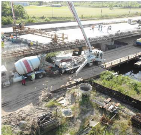
The project consists of 8.5 miles of road widening and relocation on SR 133 in Colquitt County. This Bridge is 450 feet long with 30-foot approach slabs on both sides over the Okapilco Creek North of Moultrie. Images taken by District 4 UAS Pilot Courtney Joseph Peugh.
