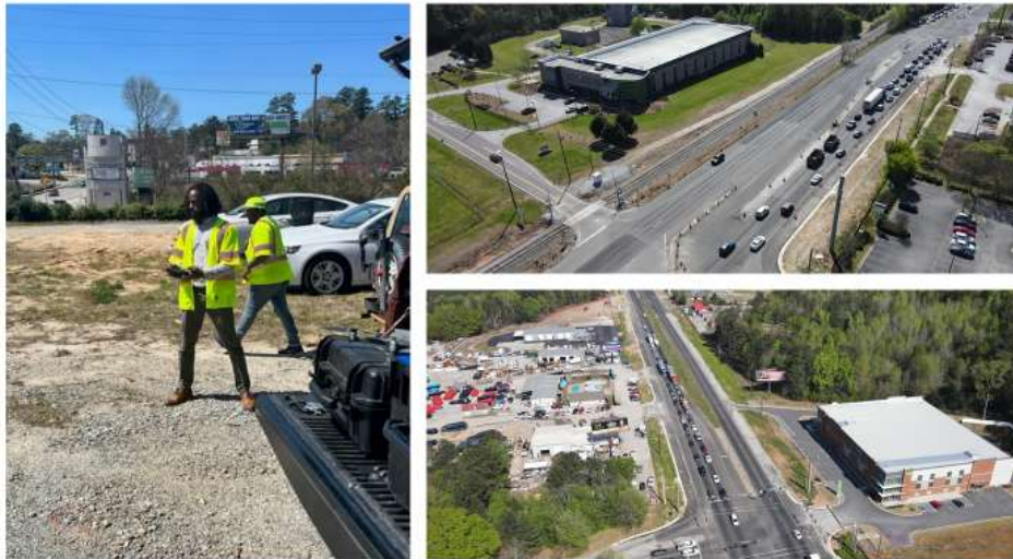
The project consists of widening SR 3US/ 19/ US 41 from an existing four-lane rural typical to a six-lane urban typical. This will include the construction of a 10-foot shared use path. Once completed the proposed project will help improve both operations and safety for the travelling public. The expected date of completion is June of 2024. Image taken by District 7 UAS Pilot Landon Pery.
