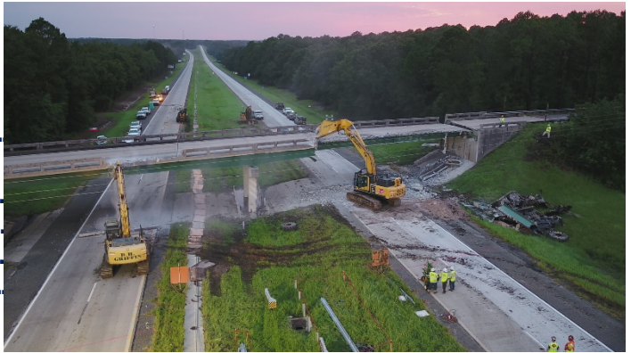
I-16 Overpass Bridge at MM 77 hit by dump truck on 7/15/21-Photo by Josh Woodard
