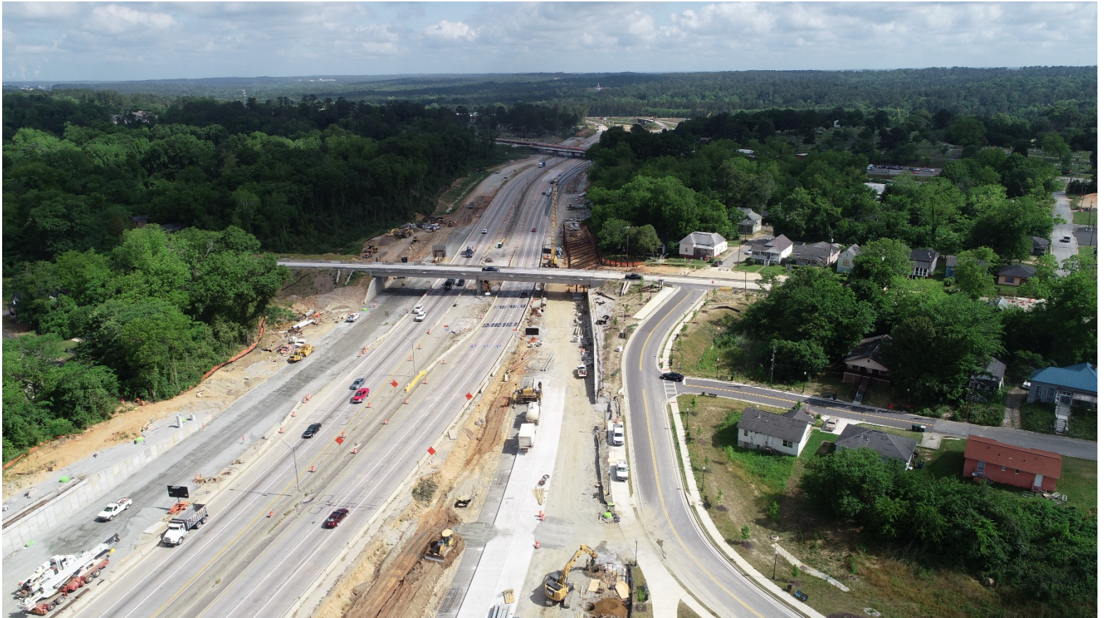
I-16 & I-75 Intersection Project
