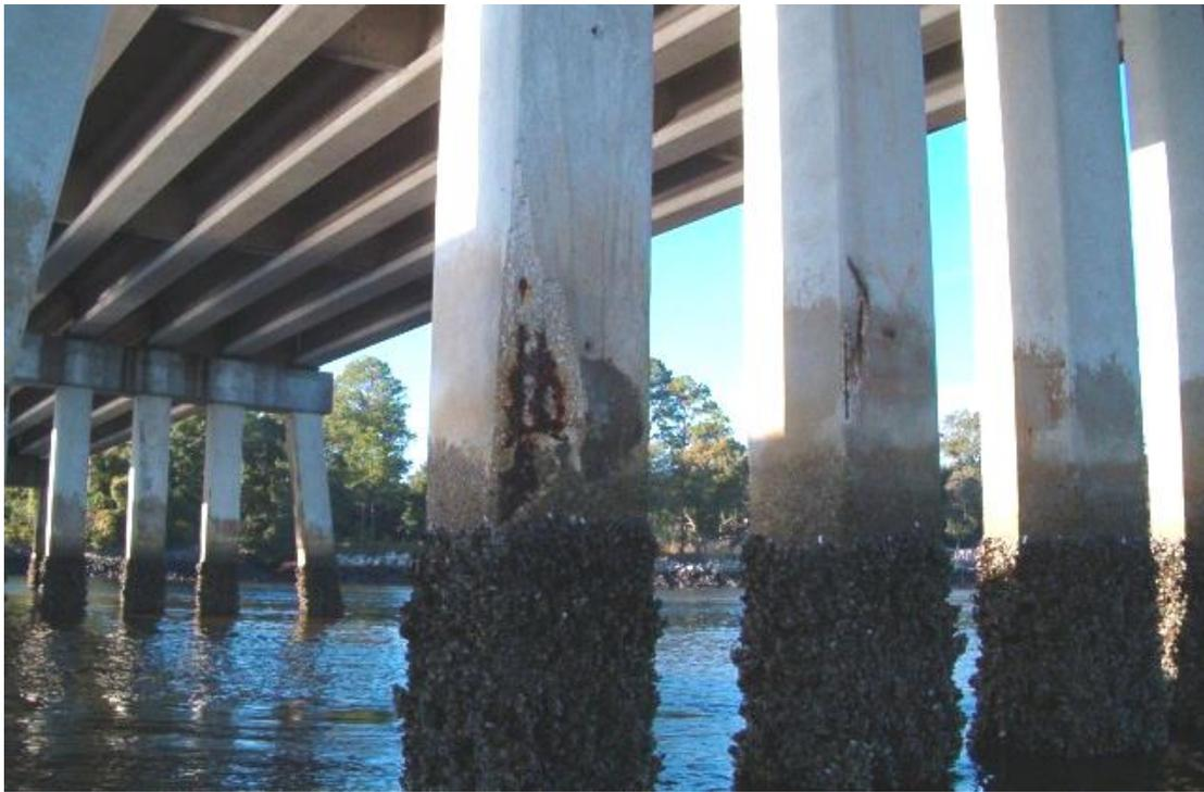
Figure 1.2 Spalling of cover concrete in splash zone of PSC piling caused by corrosion of prestressing strand and ties. Location: I-95 over the Turtle River in Brunswick, GA
