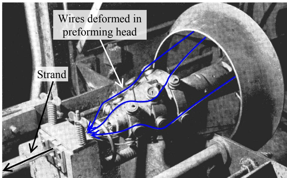
Figure 7.8 Typical preforming head (adapted from (Anderson, 1964))
