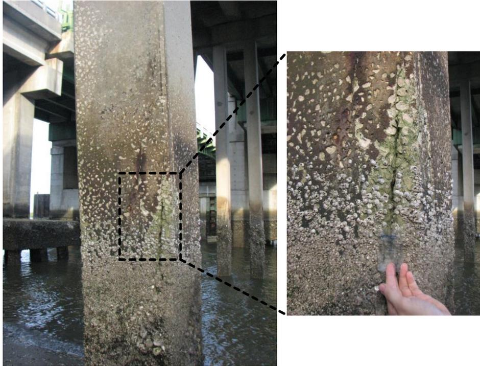
Figure 2.16 Cracks and rust staining on precast PSC piling in coastal bridge substructure.
