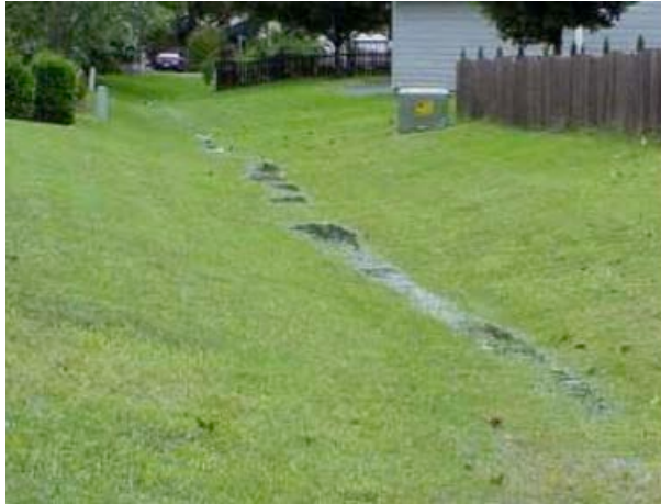
Figure 11. Grass swale. (Georgia Stormwater Manual).
