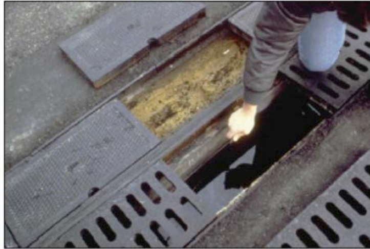
Figure 7. Perimeter sand filter (Georgia Stormwater Manual).
