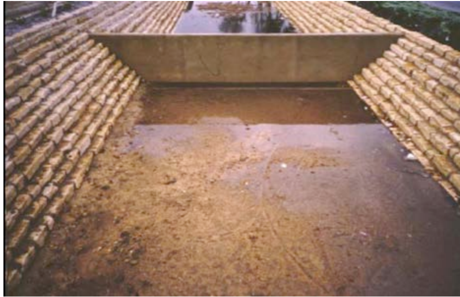
Figure 9. Newly constructed bioretention area (Georgia Stormwater Manual).
