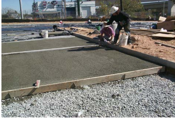
Figure 12. Porous concrete installation (Georgia Stormwater Manual).
