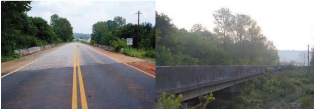
Figure B. 9 Skew T-Beam Bridge (ID: 015-0108, Bartow County)
