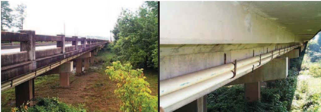
Figure B.8 Straight T-Beam Bridge (ID: 129-0045, Gordon County)
