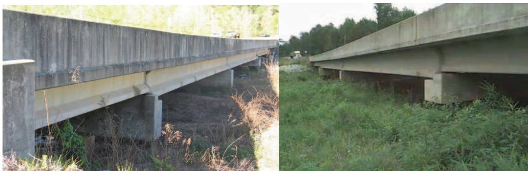
Figure B. 10 Pre-Stress Bridges (ID: 223-0034, Paulding County)
