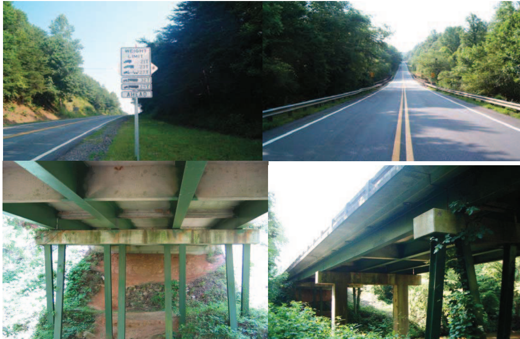
Figure B. 11 Steel Girder Bridge (ID: 085-0018, Dawson County)
