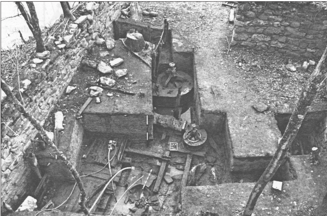
Figure 21. Photographs of Excavations at Parks Mill Showing Turbines (from Wood 1992b)
