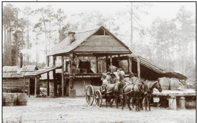
Turpentine still in Thomas County, ca. 1895. Gum brought from the woods was distilled into turpentine and rosin. The barrels were used to store the naval stores. Courtesy, Georgia Department of Archives and History.
