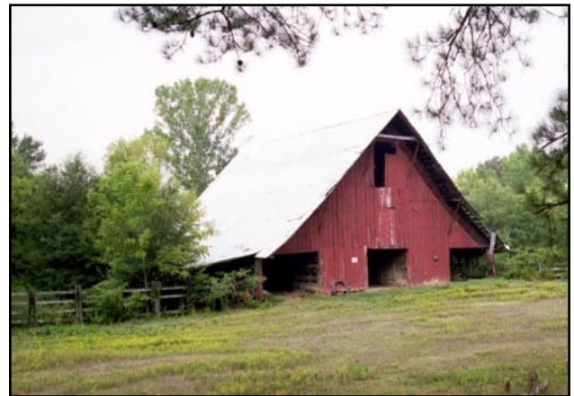
This three-portal barn in Chattooga County (Ridge and Valley Region) was historically used for mules.
