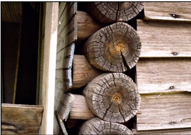
The saddle-notched corner on this log outbuilding is partially covered by weatherboard siding.
