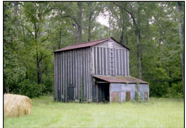
The photograph above shows a 1920s flue-cured tobacco barn in Effingham County with an attached shelter for the exterior furnace. The photograph below is a tobacco barn in Berrien County with wide overhanging sheds (shade skirts) for the stripping process. Both are located in the Central Coastal Plain.
