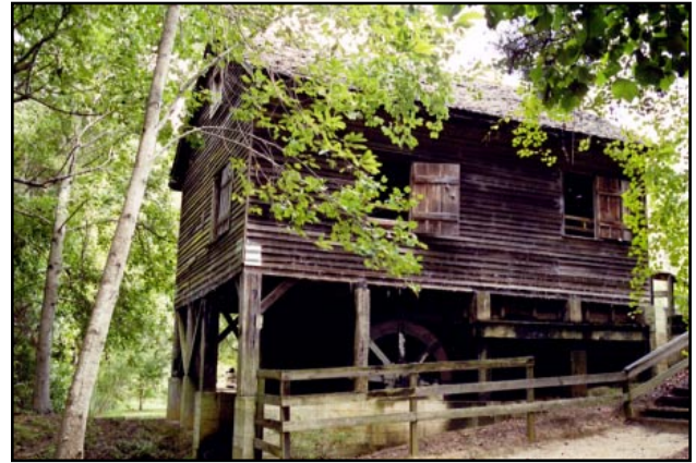
This 1879 grist mill was originally built in Worth County (Central Coastal Plain Region), and re-located to the Georgia Agrirama in Tifton.
