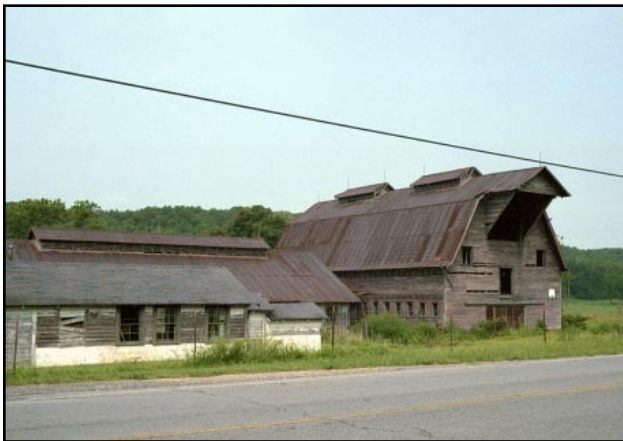
A large Appalachian barn in Murray County (Ridge and Valley Region) has a gambrel roof topped with small monitors (possibly for ventilation), and a projecting hay hood.
