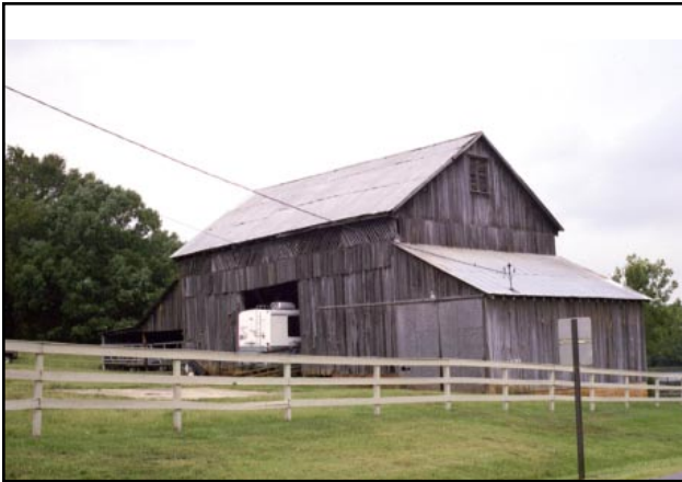
This English barn with gable-end additions in Floyd County (Ridge and Valley Region) is currently being used as a horse barn.
