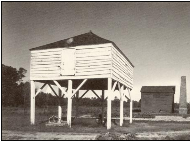
This winnowing house at Mansfield Plantation in South Carolina, and the steam-powered rice mill behind it, are examples of rarely preserved structures associated with the rice plantations of the coastal region. Source: Vlach (1993).
