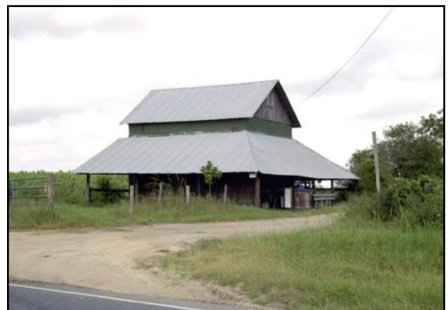
The photograph above shows a 1920s flue-cured tobacco barn in Effingham County with an attached shelter for the exterior furnace. The photograph below is a tobacco barn in Berrien County with wide overhanging sheds (shade skirts) for the stripping process. Both are located in the Central Coastal Plain.
