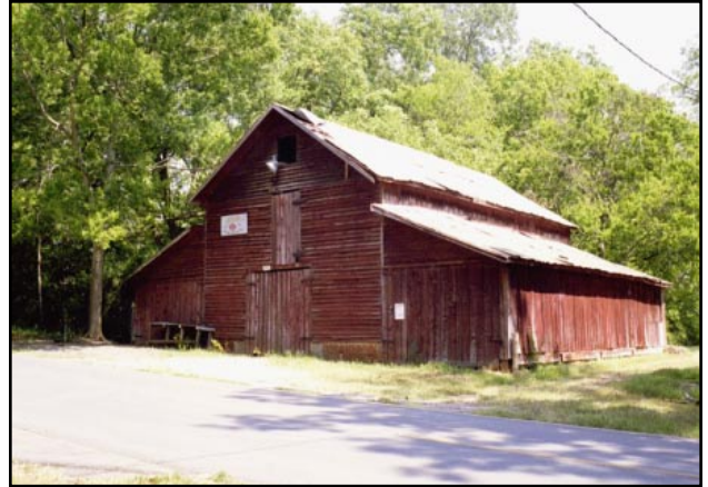
This transverse crib barn in Jones County (Piedmont Region) has flanking enclosed sheds.
