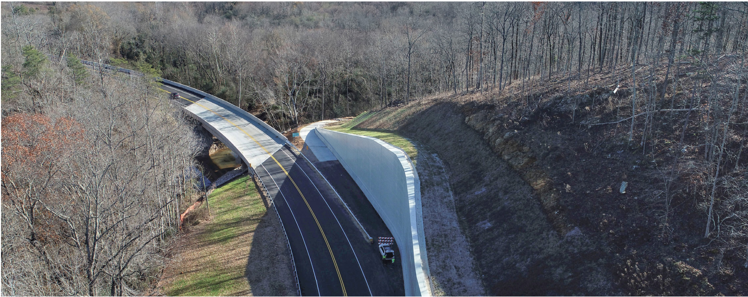
New Highway 120 bridge. Retaining wall is a safety feature.
