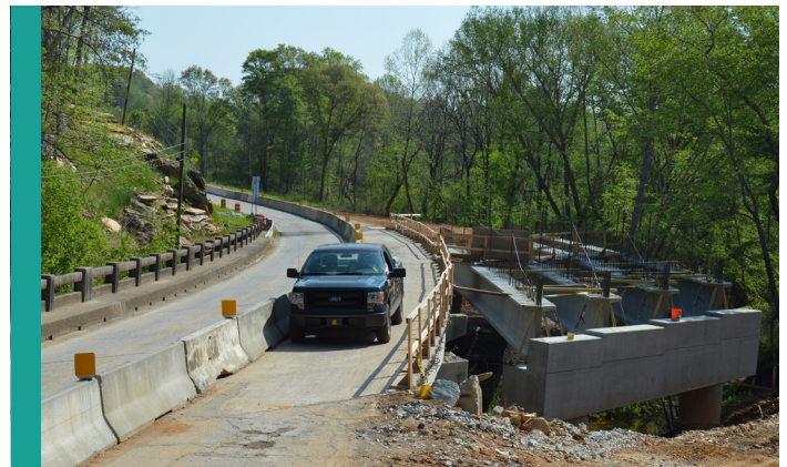
Highway 120 replacement bridge under construction to the right of old bridge.
