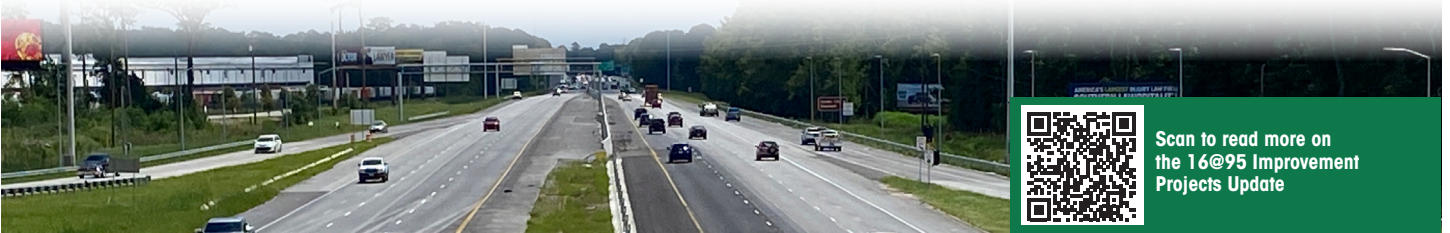
Top Photo: I-95 northbound view at bridge over I-16
