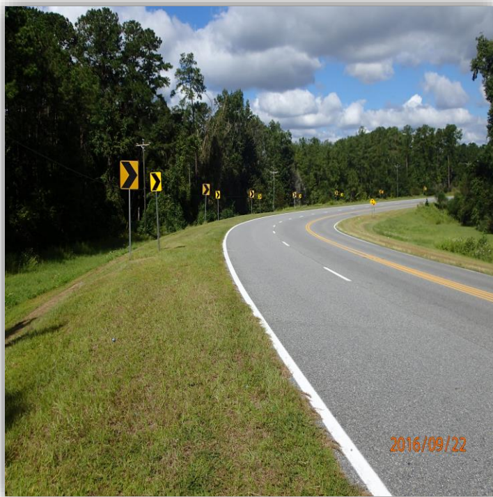
Lowndes County - New advanced sharp curve signs on Val-Tech Road
