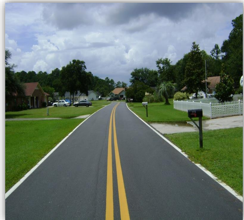
St. Mary's – New centerline and edge line striping on Cambray Circle.
