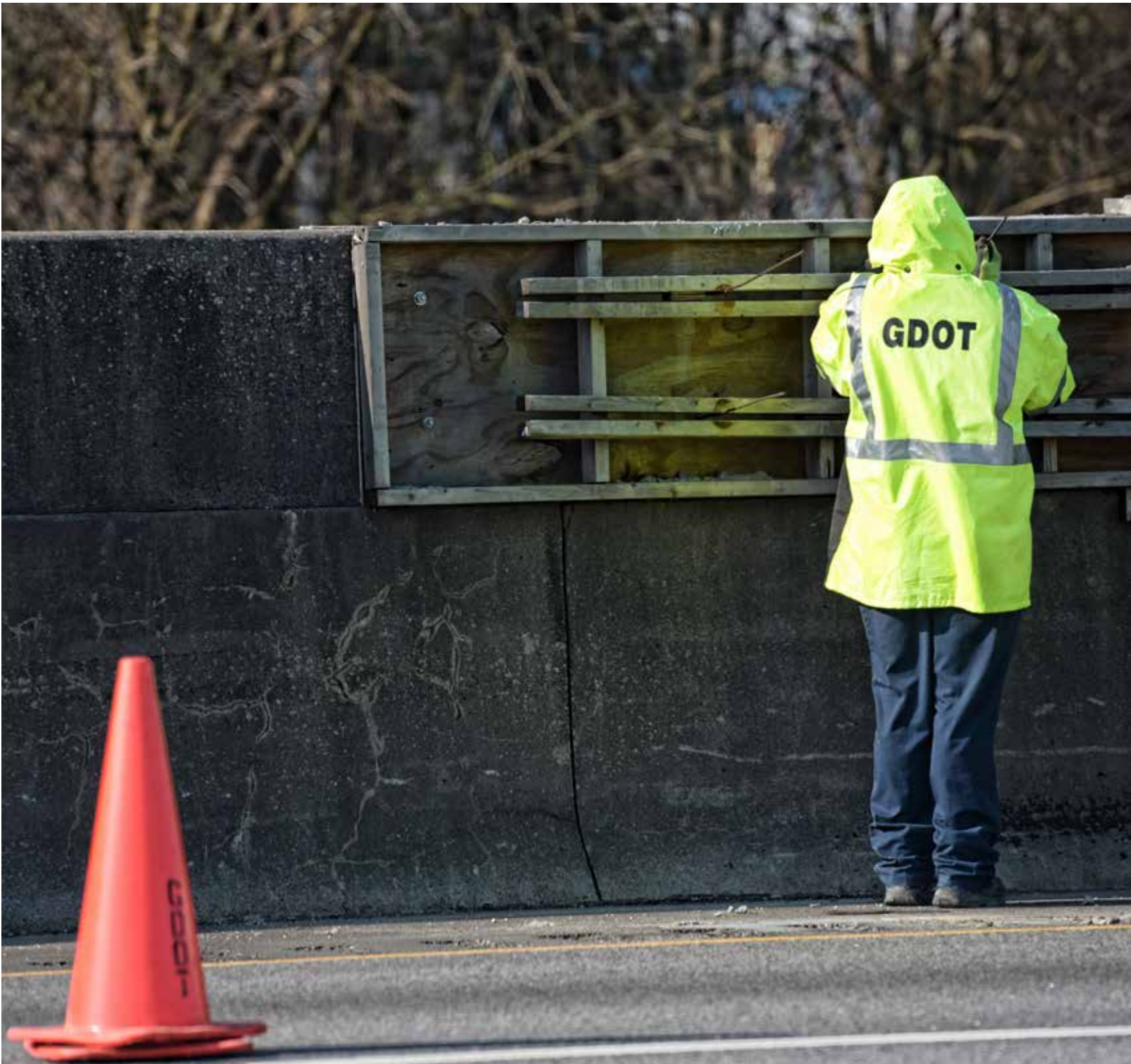
Repairing a concrete barrier wall. Photo: Cedric Mohr, GDOT
