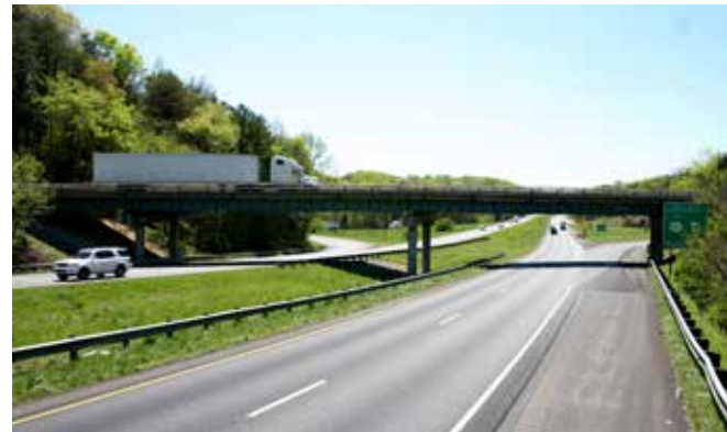
The 51-year old SR 299 Bridge will be replaced using accelerated bridge construction technology. Photo: David Sullivan, GDOT
