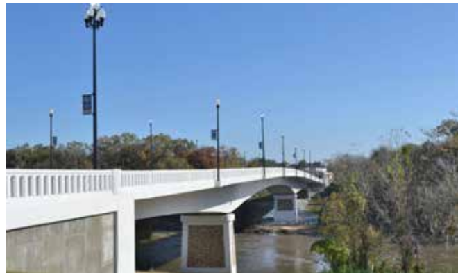
Albany's Broad Avenue Memorial Bridge features unique construction, long archways, decorative lighting and masonry inlaid piers. Photo: Nita Birmingham, GDOT
