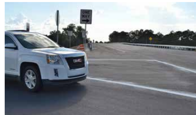
View at the top of the I-75 North exit ramp in 2014. The narrow bridge and the proximity of the ramp made it difficult to see oncoming traffic.
