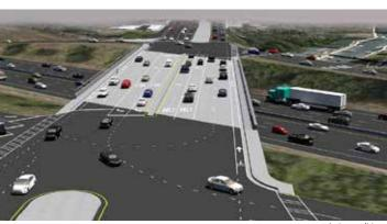
About the project. With the population growth in DeKalb County, the I-285 at Flat Shoals Bridge Reconstruction project is designed to improve the safety and efficiency of the interchange with two through lanes in each direction, bike lanes on both sides, and dual left-turn lanes from SR 155 NB and SR onto I-285 FB and WB. The interstate exit will be widened with dual left-turn and dual right-turn lanes onto SR 155/ Flat Shoals
