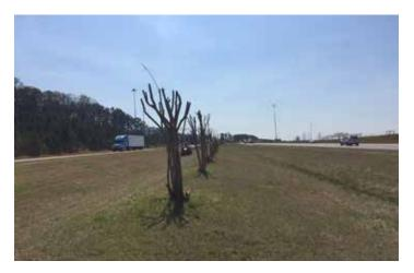
**Bioswales.** The Ray and the Georgia Department of Transportation installed five acres of native grasses and pollinator plant seeds in the median and northbound lane gore area of Exit 6 on I-85 near LaGrange. These areas, known as bioswales, are shallow drainage ditches filled with vegetation to slow water movements and capture particulate pollutants, heavy metals, rubber and oil during rainstorms. Photo: The Ray
