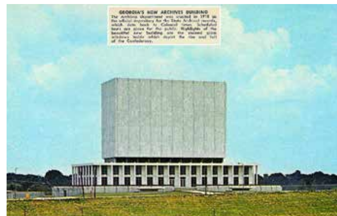
Georgia Archives Building, built in 1965, was District 7's temporary home from 2004 to 2007 when the Chamblee location was undergoing renovation. The building, which had structural issues, was demolished in March. Postcard image: Atlanta Time Machine
