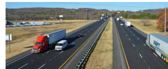
Newly resurfaced I-95 in Catoosa and Whitfield counties. Photo: David Sullivan, GDOT
