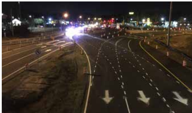
The new $6.3 million DDI in Chatham County is Georgia's first diverging diamond interchange outside Metro Atlanta. It is also the state's first DDI featuring an interstate off-ramp with triple-left turn capability. Photo: Jill Nagel, GDOT
