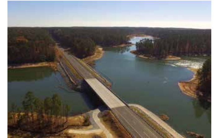
Keg Creek Bridge. Photo: Larry Morris, GDOT
