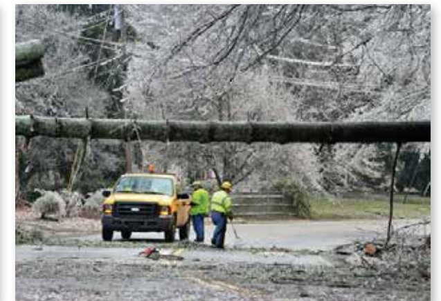
Clearing trees downed from a winter storm
