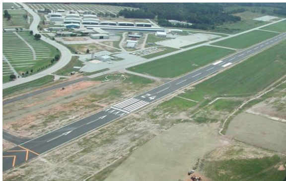
Hampton - Atlanta South Regional Runway Extension - $3,044,664
