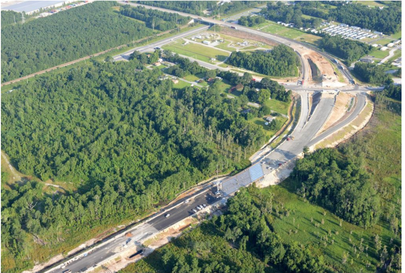
Jimmy Deloach Connector at Sonny Dixon Interchange, Chatham County
