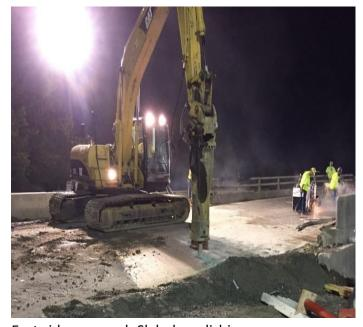
East side approach Slab demolishing
