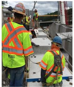
Setting of Pre-Cast Pedestals at Bent 3
