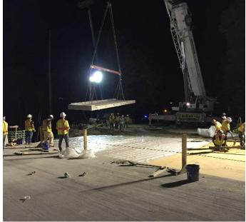
Setting of Precast Approach Slab - Bent 3
