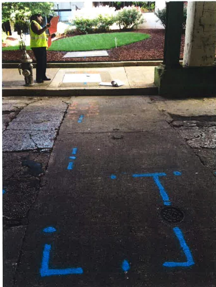
Existing Valve at +/-19+40 Collins Street
