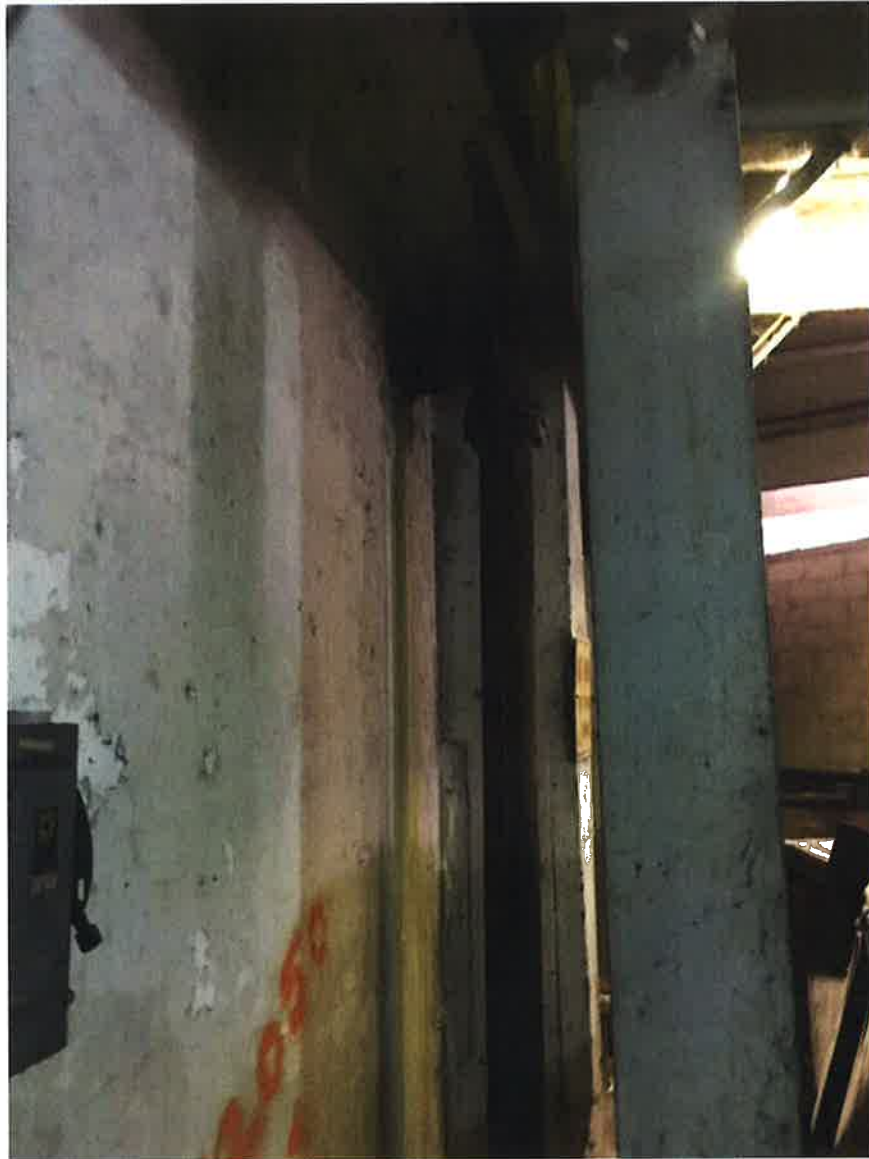
Existing water main riser +/- Sta 24+50 Collins Street
