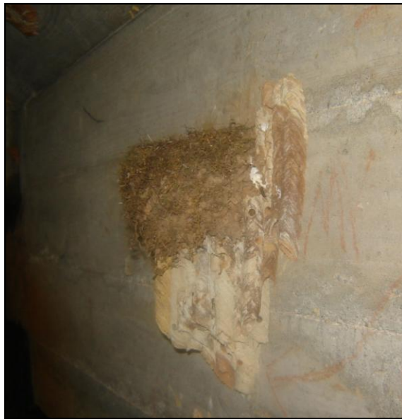
Eastern phoebe nest under a bridge
