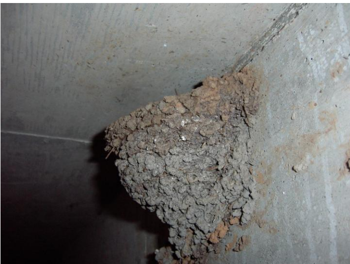
Barn Swallow nest under a bridge.
