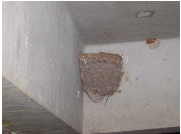
Barn Swallow nest under a bridge.
