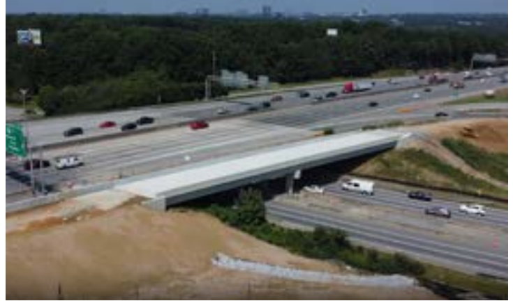
I-285/Peachtree Boulevard Interchange Improvements Project, Doraville, Georgia
