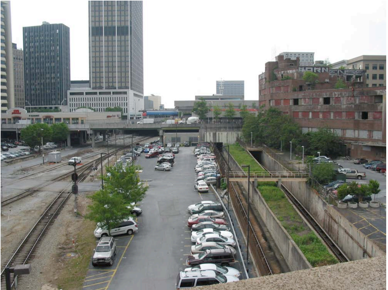
Figure 4-12 The Site of the Proposed MMPT Showing the existing NS and CSX Tracks on the Left and the MARTA Lines (in the Trenches) on the Right
