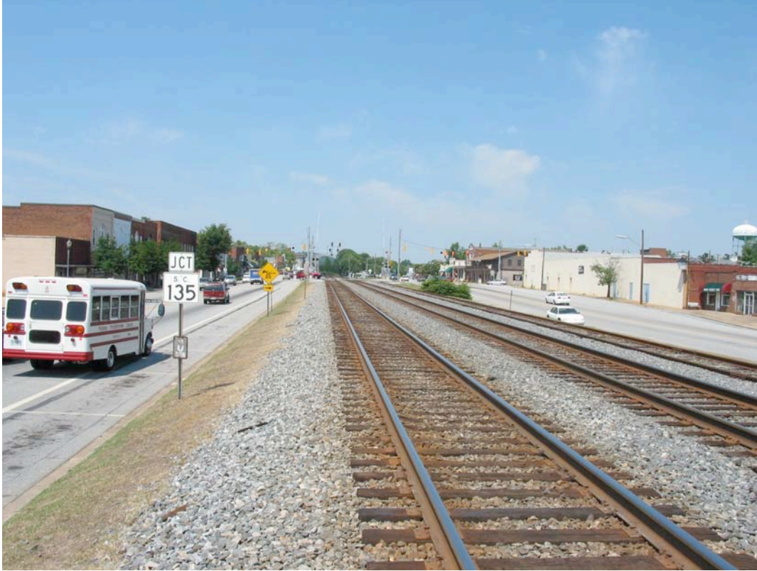
Figure 4-6 Double Track and Siding on Route 135 in South Carolina
