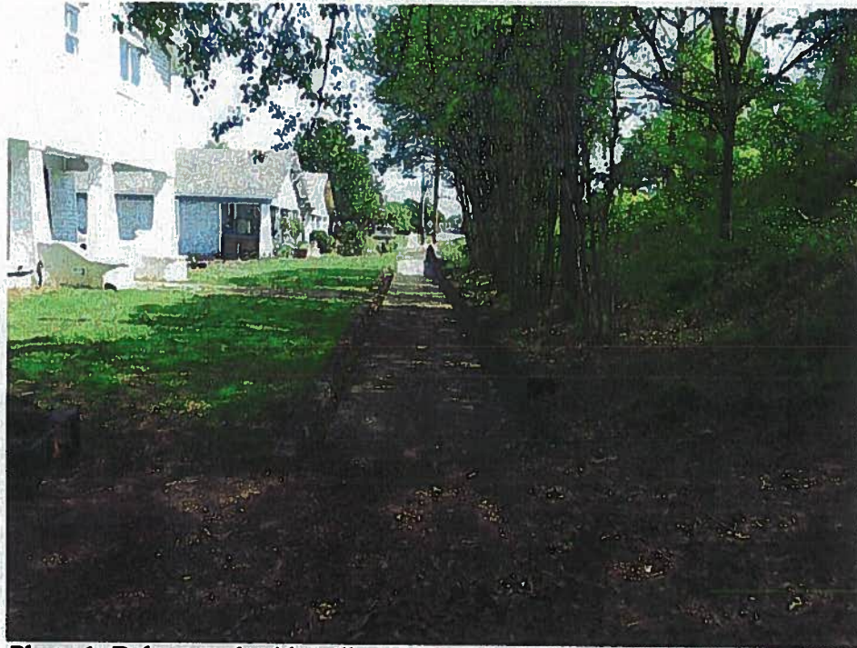
Photo 1: Below grade sidewalk at 301, 305, and 315 South Cherokee Road, looking north.
