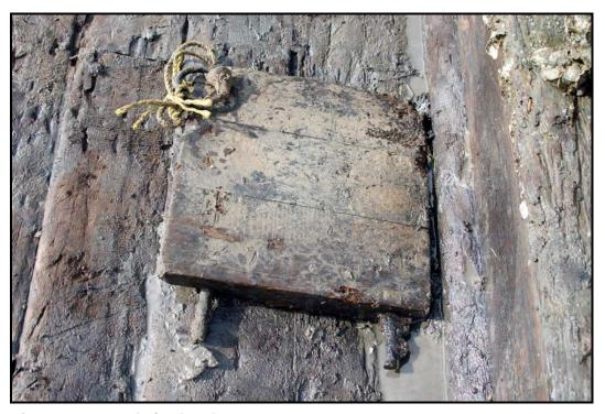
Figure 66. Hatch for lumber port.
