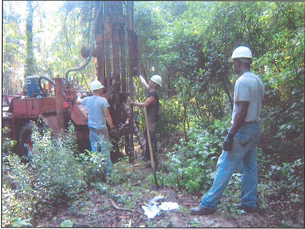
Figure 23. Boring activities on Trellis property.
