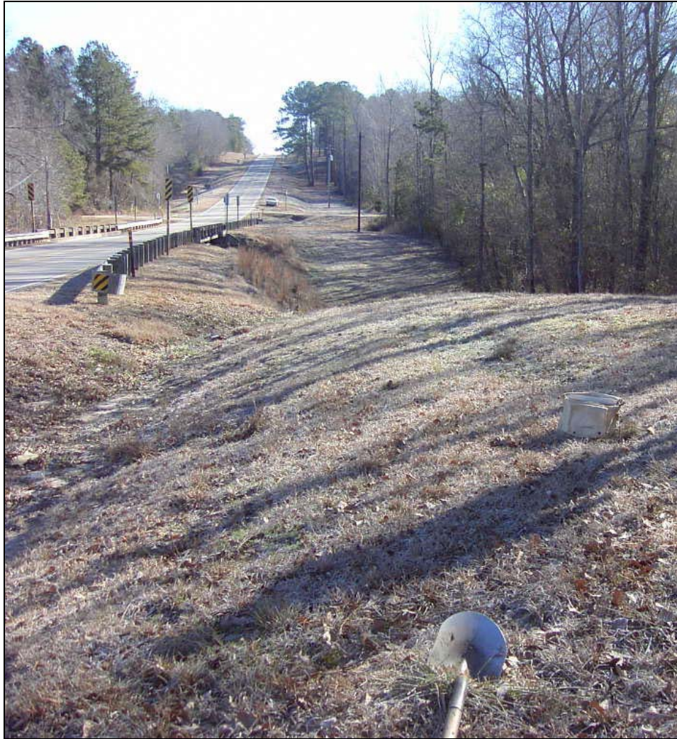
Figure 8. General Area Around Unit 2; South Side of SR 102 Looking East.
