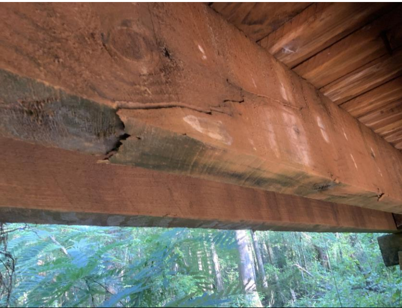
Cracking
