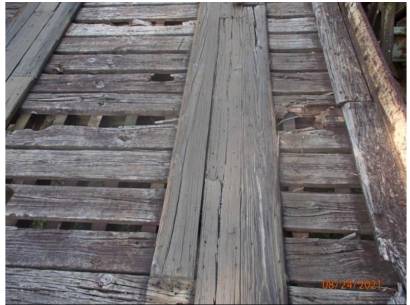
Missing/Deteriorated Boards
