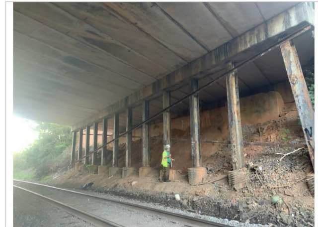
Underneath looking at bent 3. 2022
