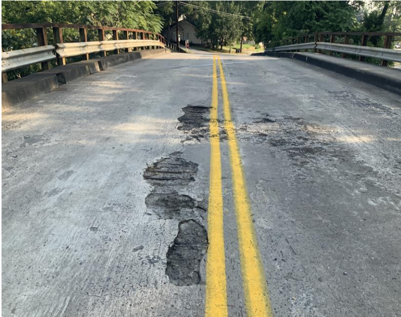
Spalls/Delamination
