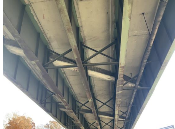
Paint Failure
