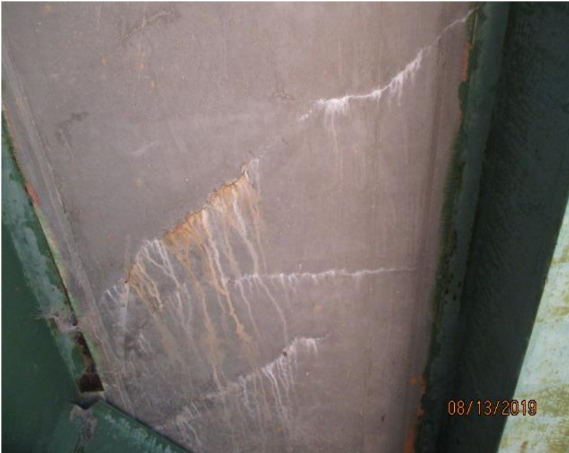
Efflorescence
