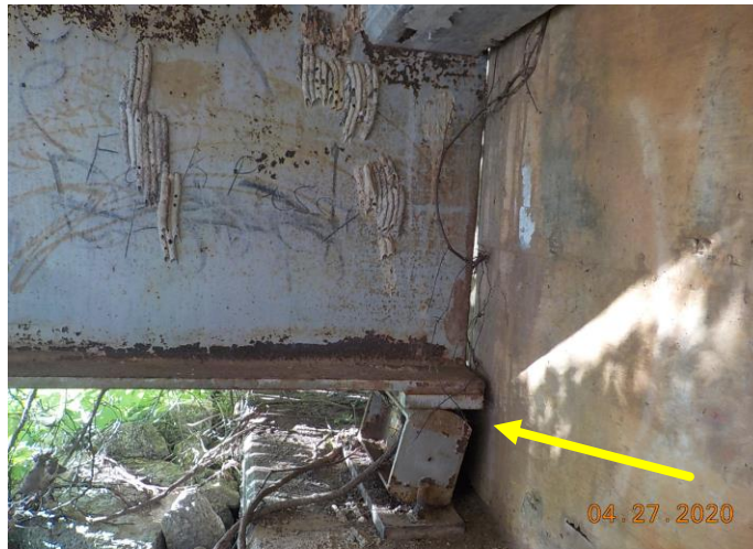
Bearing Misalignment
