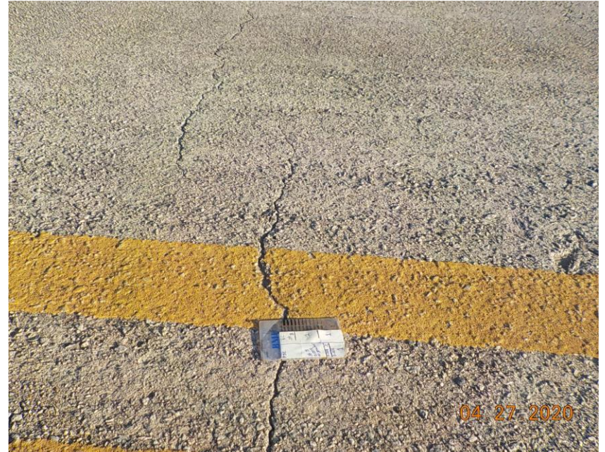
Cracking
