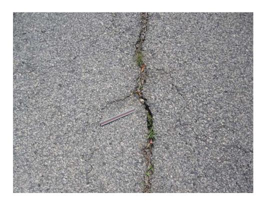
A01LW-50. Longitudinal and Transverse Cracking (Sample Unit #01).
