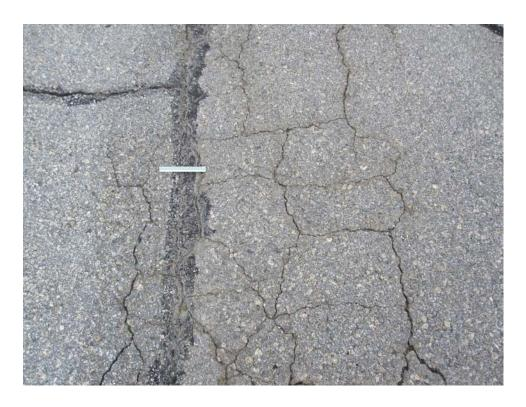
THLW-20. Alligator Cracking (Sample Unit #03).
