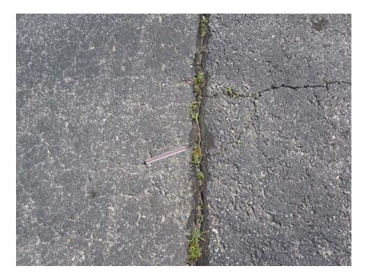
A02LW-10. Longitudinal and Transverse Cracking (Sample Unit #10).
