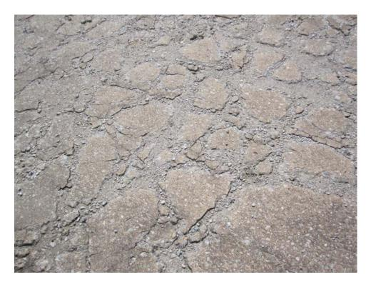
A01LW-40. Shattered Slab (Sample Unit #04).
