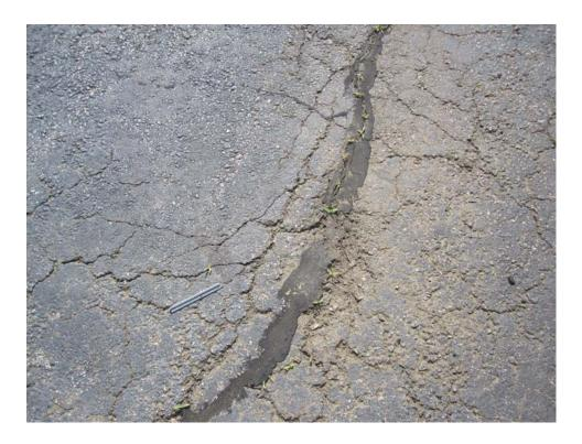
A02LW-10. Alligator Cracking (Sample Unit #10).
