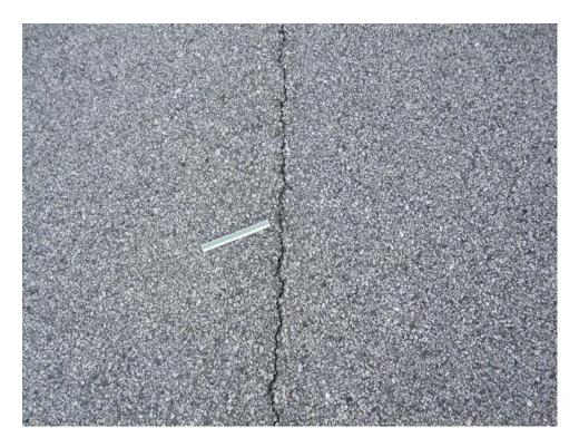
$TZLW\hbox{-}20.\ Longitudinal\ and\ Transverse\ Cracking\ (Sample\ Unit\ \#03).$
