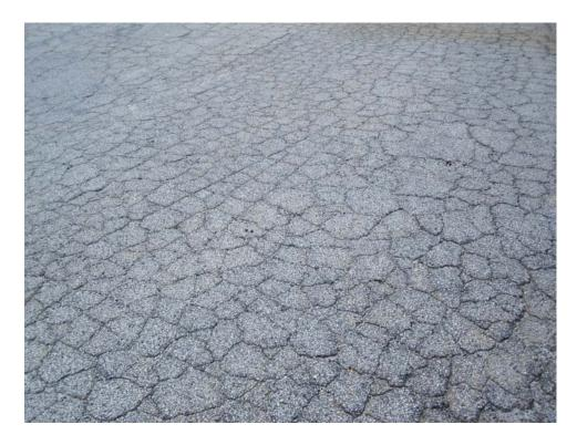
A01LW-30. Alligator Cracking (Sample Unit #02).
