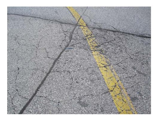
TDLW-10. Rutting and Alligator Cracking (Sample Unit #01).
