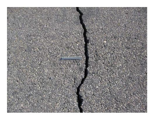
TBLW-10. Longitudinal and Transverse Cracking (Sample Unit #03).
