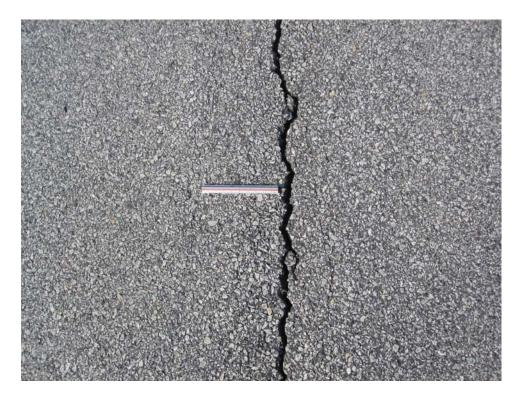
TWLW-30. Longitudinal and Transverse Cracking (Sample Unit #06).
