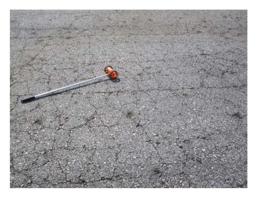
A04LW-10. Alligator Cracking (Sample Unit #03).
