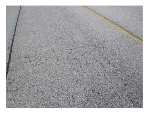
TWLW-10. Alligator Cracking (Sample Unit #09).
