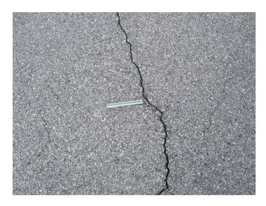
A01LW-60. Longitudinal and Transverse Cracking (Sample Unit #07).
