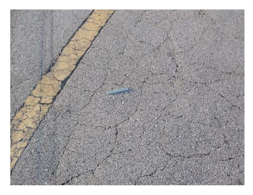
TCLW-10. Alligator Cracking (Sample Unit #04).
