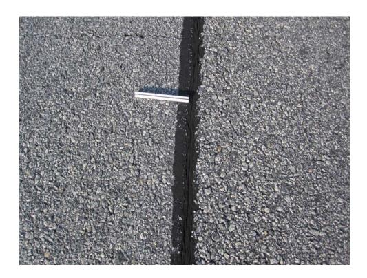
TWLW-10. Longitudinal and Transverse Cracking (Sample Unit #03).
