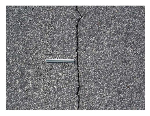
A04LW-20. Longitudinal and Transverse Cracking (Sample Unit #01).
