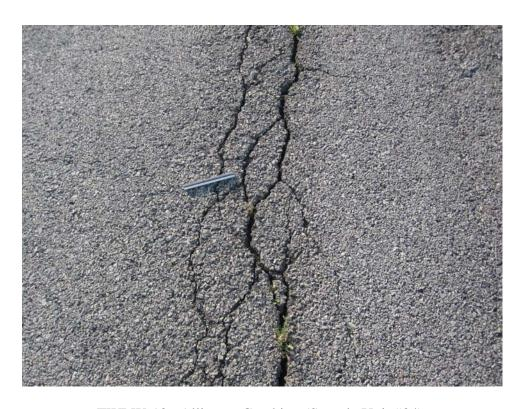
TWLW-10. Alligator Cracking (Sample Unit #04).
