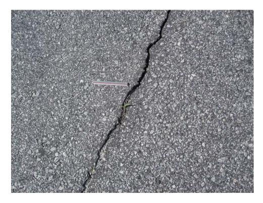
A02LW-20. Longitudinal and Transverse Cracking (Sample Unit #25).
