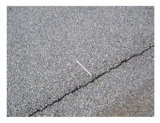
TZLW-10. Longitudinal and Transverse Cracking (Sample Unit #03).
