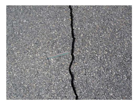
TELW-10. Longitudinal and Transverse Cracking (Sample Unit #01).
