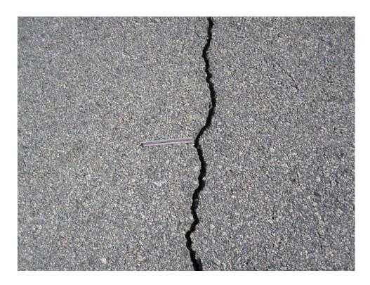
TGLW-10. Longitudinal and Transverse Cracking (Sample Unit #01).
