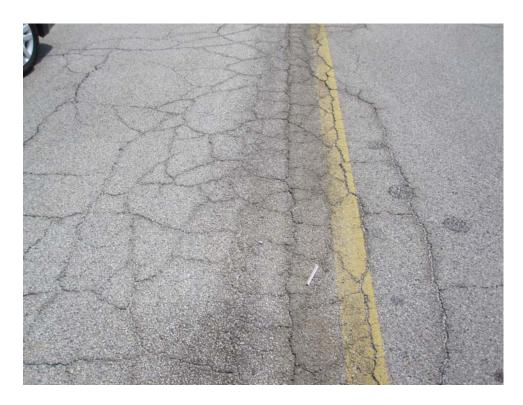
A01LW-60. Alligator Cracking (Sample Unit #05).
