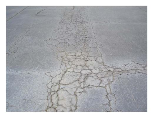
A03LW-10. Alligator Cracking (Sample Unit #11).
