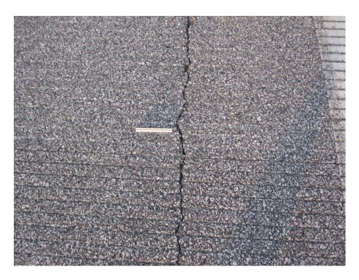
$R725LW\text{-}10. \ \ Longitudinal \ and \ Transverse \ Cracking \ (Sample \ Unit \ \#117).$
