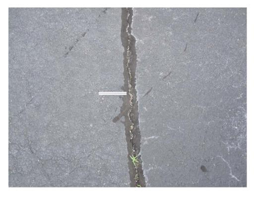
A03LW-10. Longitudinal and Transverse Cracking (Sample Unit #22).
