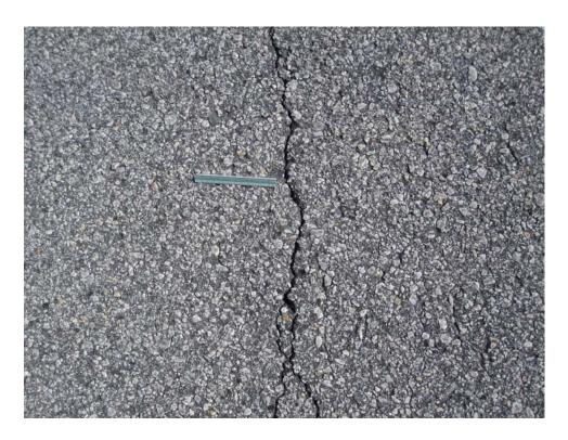
TDLW-10. Longitudinal and Transverse Cracking (Sample Unit #01).
