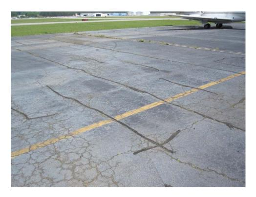
A03LW-20. Alligator and Block Cracking (Sample Unit #26).
