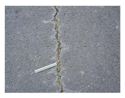
A01LW-20. Longitudinal and Transverse Cracking (Sample Unit #35).
