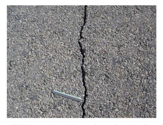
TFLW-10. Longitudinal and Transverse Cracking (Sample Unit #01).
