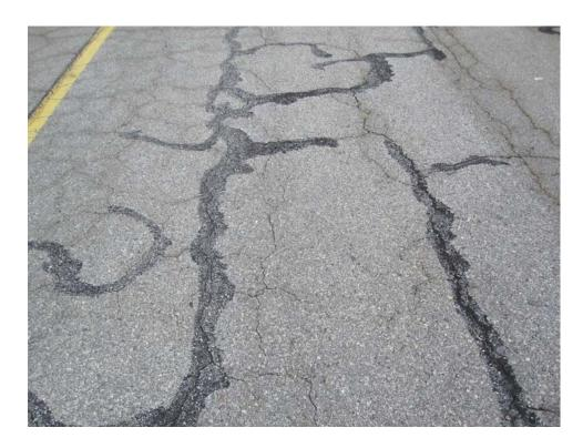
THLW-20. Block Cracking (Sample Unit #01).
