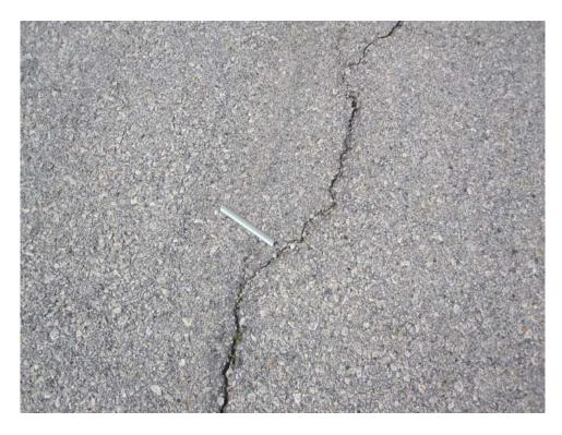
A01LW-10. Longitudinal and Transverse Cracking (Sample Unit #12).
