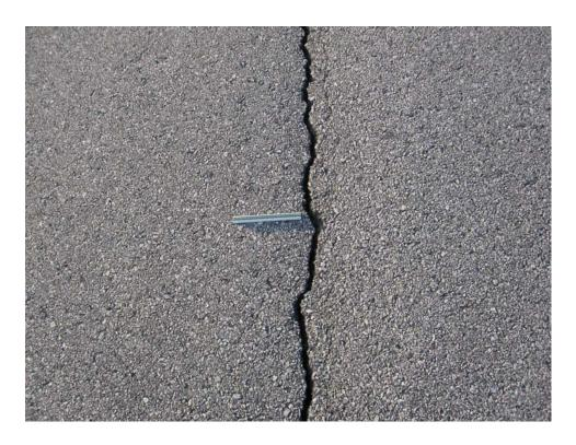
TCLW-10. Longitudinal and Transverse Cracking (Sample Unit #02).
