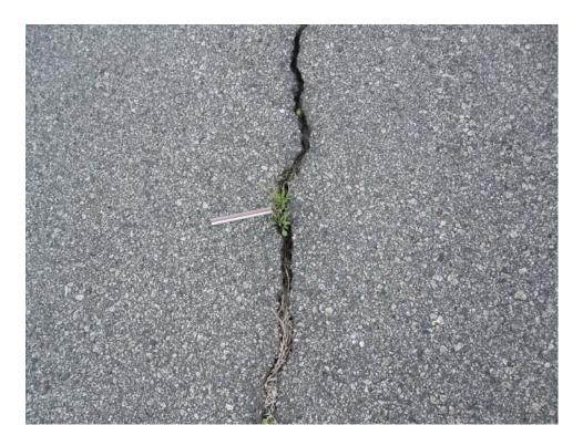
A03LW-20. Longitudinal and Transverse Cracking (Sample Unit #06).
