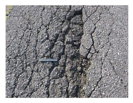
TBLW-10. Alligator Cracking (Sample Unit #01).
