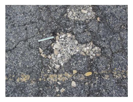
A01LW-70. Alligator Cracking (Sample Unit #03).
