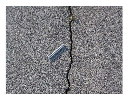
$TWLW\mbox{-}20. \ \ Longitudinal \ and \ Transverse \ Cracking \ (Sample \ Unit \ \#02).$
