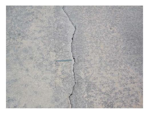
THANGLW-10. LTD Cracking (Sample Unit #04).
