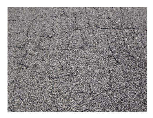
TWLW-10. Alligator Cracking (Sample Unit #51).
