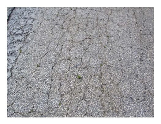
TYLW-10. Alligator Cracking (Sample Unit #20).
